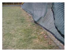
Perimeter fencings and backstops for the Mills Field ball diamond are in need of replacement. The original installation dates back to 1959. Despite numerous repairs over the years, the present condition has reached a critical level and will require total replacement. Replacement would include new and updated backstops, complete perimeter fencing with gates, and efficiency improvements to the irrigation system.
