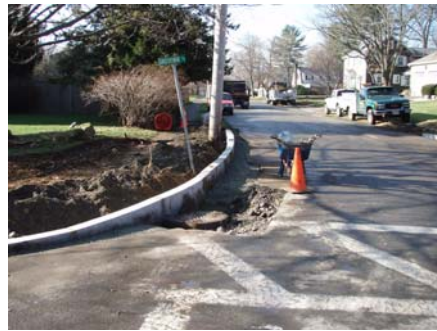
Sidewalk Repair and Resurfacing
