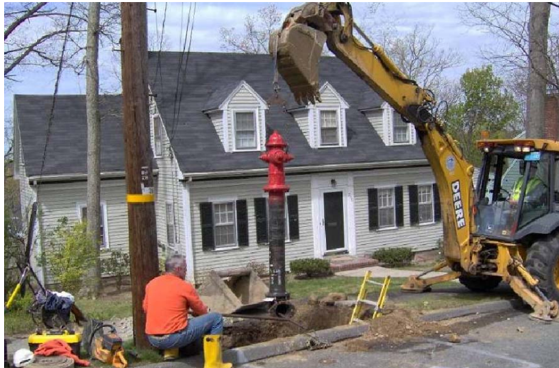
Fire Hydrant Replacement
