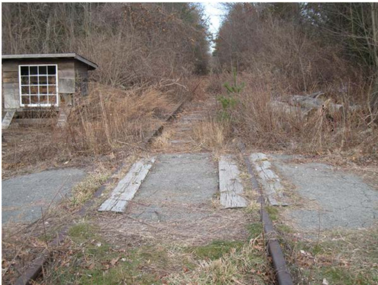
Figure 24: Existing Private Crossing
