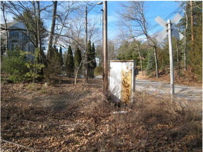
Figure 51: Charles River Street Crossing Rail Infrastructure
