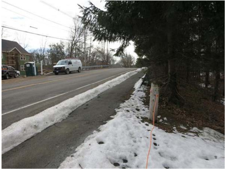
Figure 38: Existing High Rock Street Sidewalk at Town Forest Driveway
