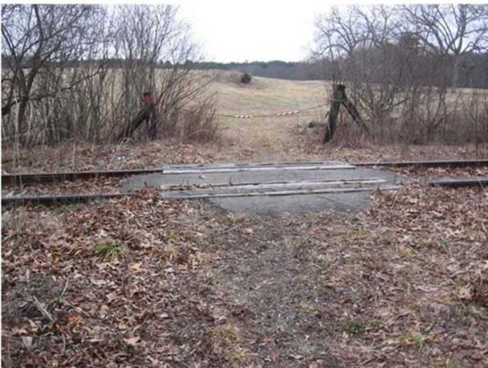
Figure 17: Private Crossing from Walker School to Charles River Peninsula
