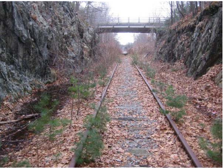
Figure 49: Existing Drainage Swales Along ROW
