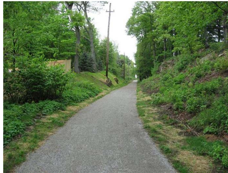
Figure 6: Example Stone Trail Surface Over Dense Graded Crushed Stone Following Construction (Topsfield Linear Common)
