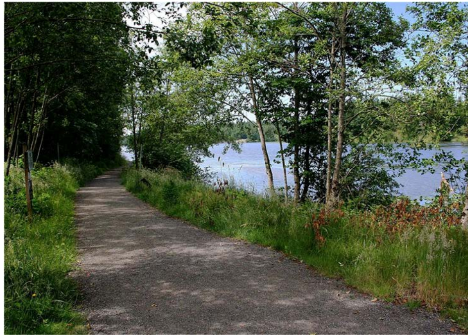
Figure 4: Example Dense Graded Crushed Stone Surface (Representative Photograph)
