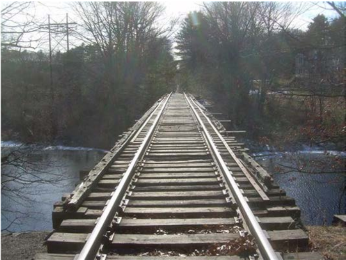
Figure 47: Charles River At Existing Timber Trestle
