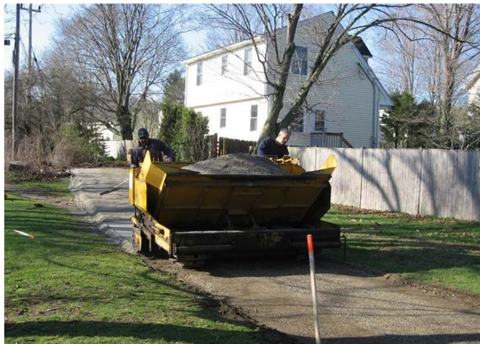
Figure 5: Example Stone Trail Surface Over Dense Graded Crushed Stone During Construction (Topsfield Linear Common)
