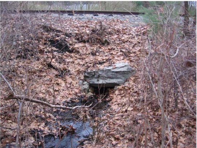
Figure 48: Existing Stream Crossing Via Culvert Under ROW
