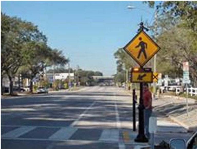
Figure 37: Example Rectangular Rapid Flashing Beacon Installation (FHWA)
