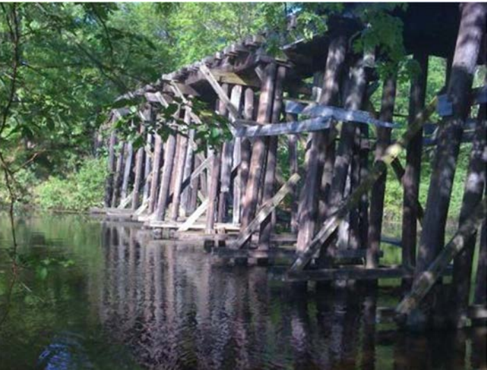
Figure 15: Existing Timber Railroad Trestle Over the Charles River
