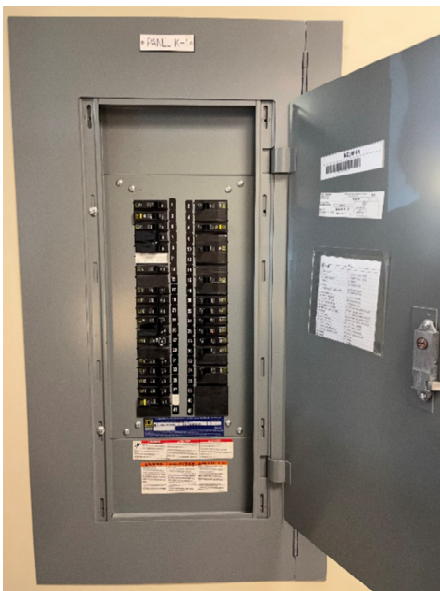
Existing Kitchen Panel
