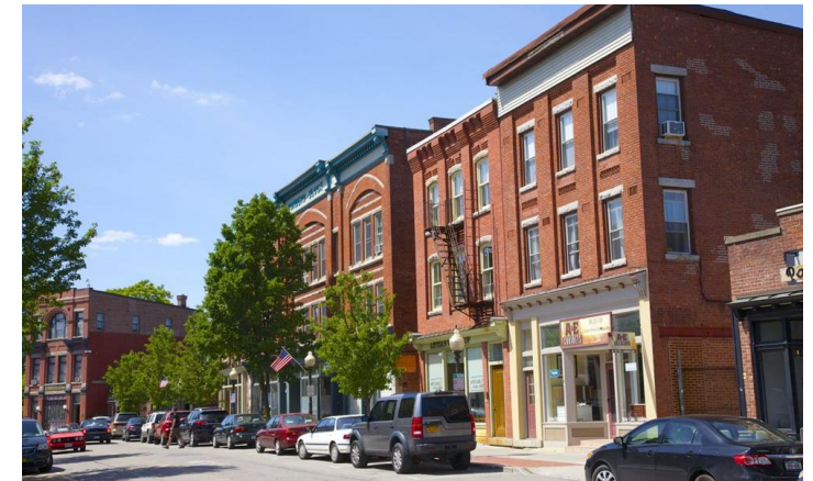
3-story MXU multifamily
