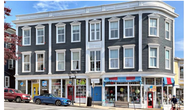
3-story MXU multifamily
