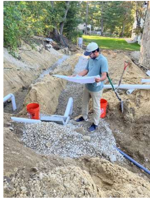
Sainath Palani, Environmental Health Agent, conducting a residential septic system installation inspection.
