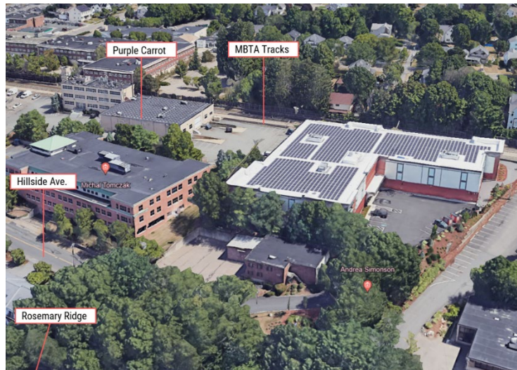
Figure 21: Hillside Industrial District – Base Compliance
