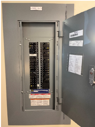
Existing Kitchen Panel
