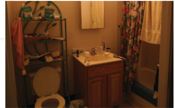
Bathrooms are worn and out of date
