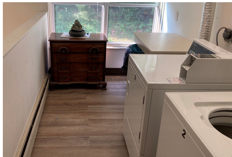
2nd floor laundryrooms are inaccessible CPA Hearing - 3/15/23
