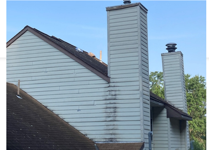
Water damage at Captain Cook Envelopes
