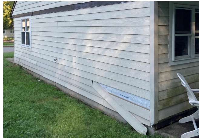
Deteriorated Siding
