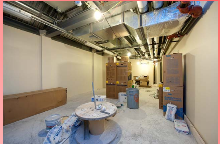
3 rd Floor Addition
