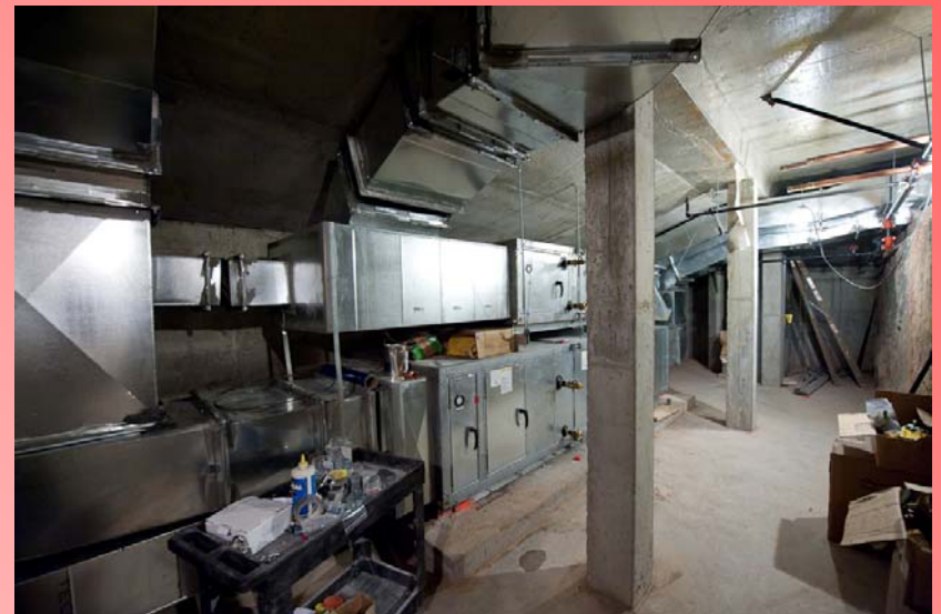
Lower Level Old Building
