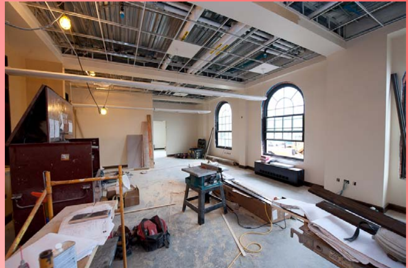
2 nd Floor New Addition
