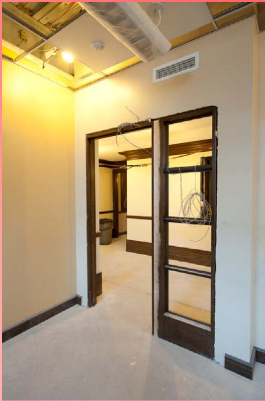
Lower Level New Addition
