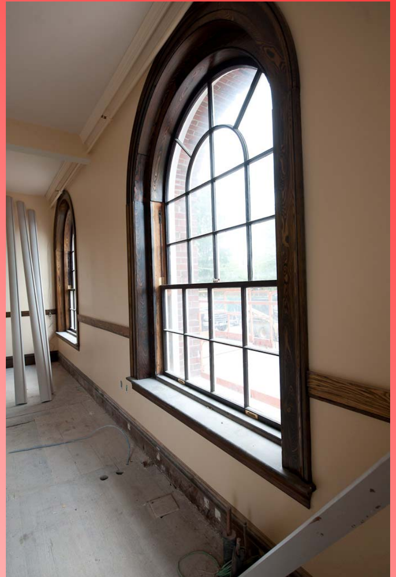
Old Building First Floor
