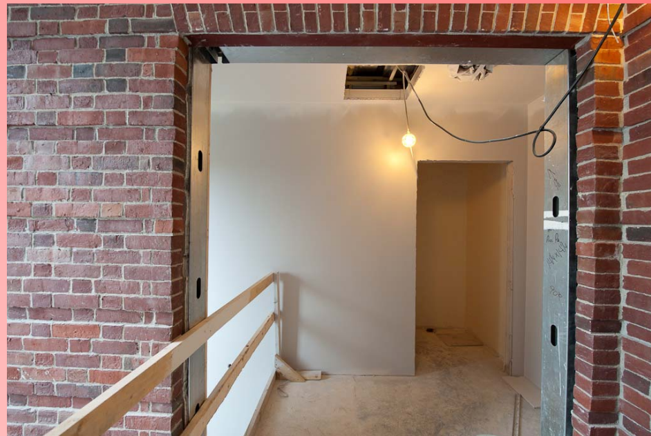
1 st Floor Addition
