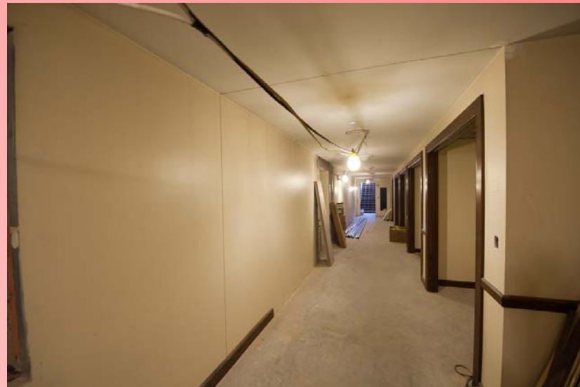
Lower Level Old Building
