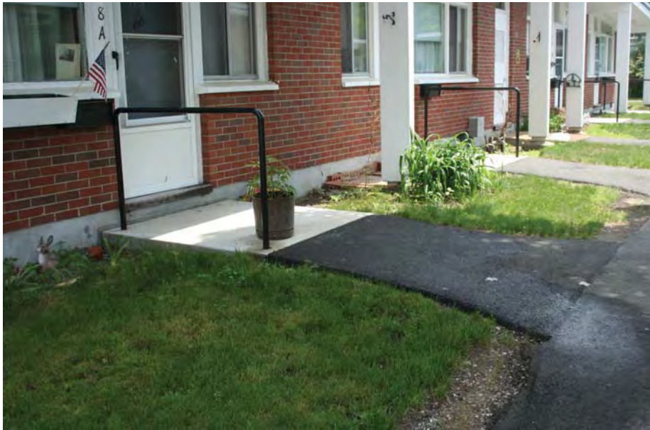
6. Some apartments have stoops at walkway level, but the first floor is still a step up so that none of the apartments are accessible or visitable (someone in a wheelchair can't visit).
