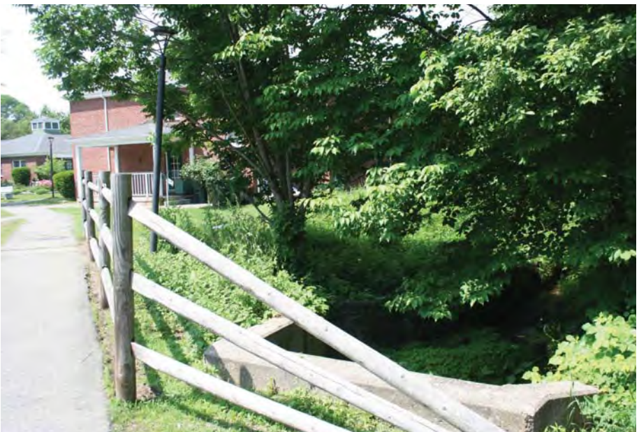
6. The entire site is relatively low and adjacent to the wetlands. Running water is culverted under the development, daylighting in three locations.
