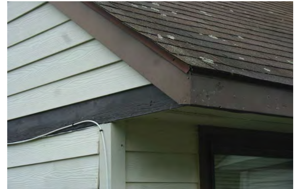
12. Roofs, eaves, soffits and trim are all in relatively poor condition. Their construction is similar to Seabeds, which suffered damage from ice dams in 2015 requiring $1.6 million dollars in emergency repair funding. The current estimate to repair Captain Robert Cook construction defects is $1.1 million.
