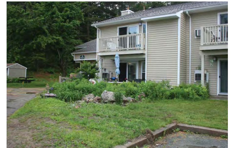
12. Roofing, siding, soffits and trim were replaced in 2015 along with underlying sheathing. The envelopes are in reasonably good condition.
