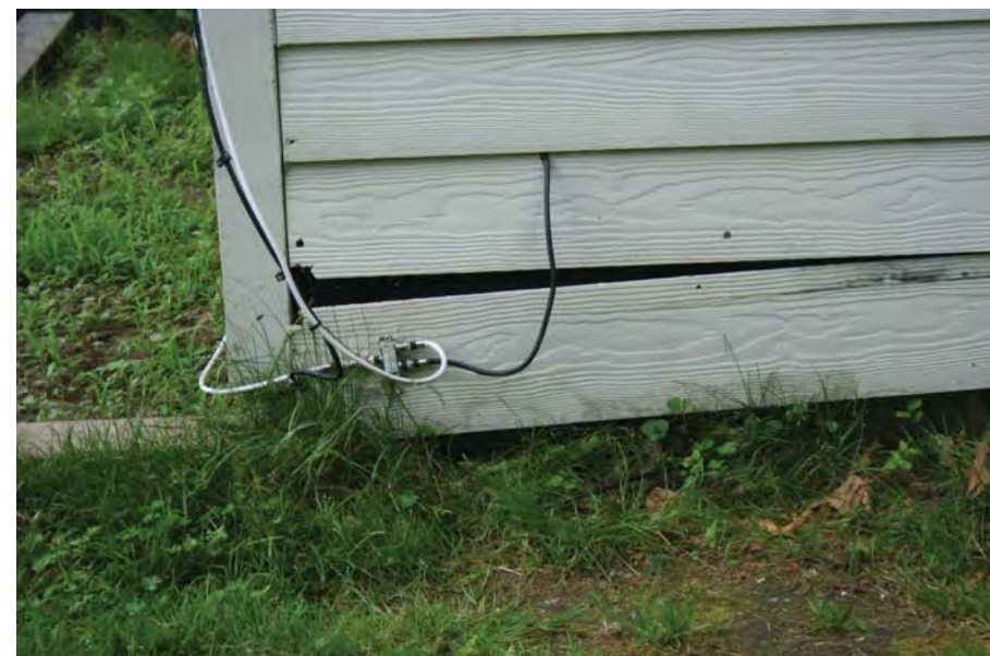
11. Siding and many of the exterior finishes appear to be near the end of their useful life. The underlying construction is of poor quality and vulnerable to deterioration and should be replaced in the near future as indicated in recent reports.
