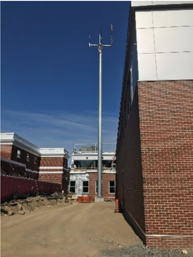
PSC 5/20 Monopole installation
