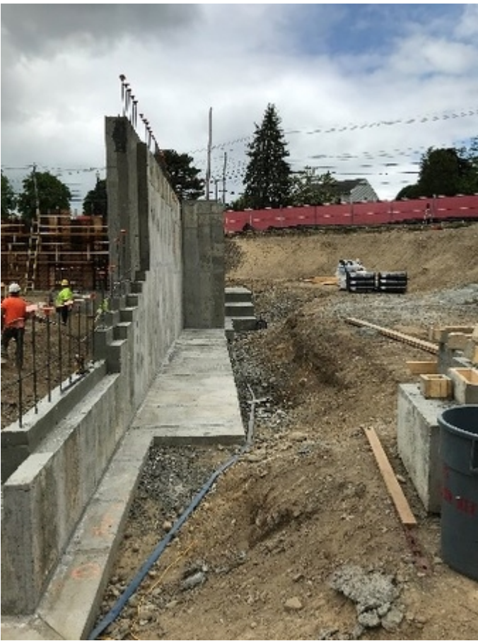
FS#2 5/20 Beginning foundations at FS#2
