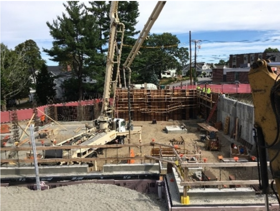
FS#2 8/20 Continuing foundation & perimeter walls
