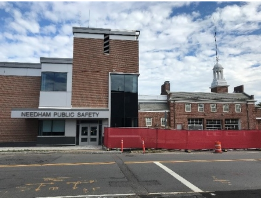
PSC 9/20 West elevation of new Public Safety entry on the left and existing old Public Safety on the right
