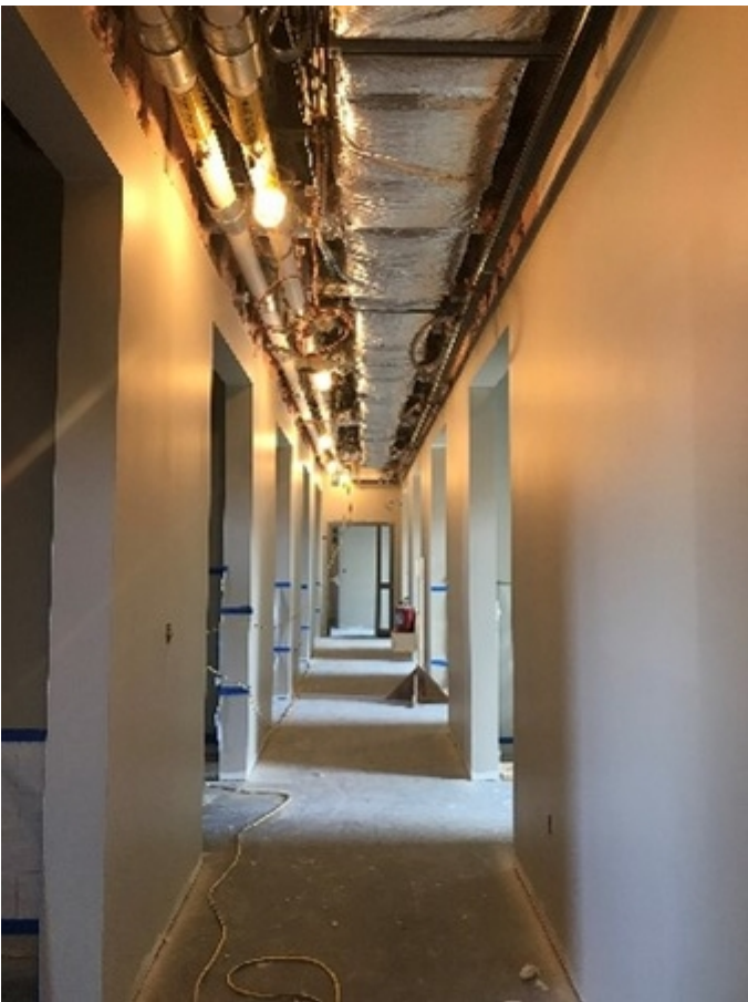
PSC 2/20 Interior finishes at bunk area
