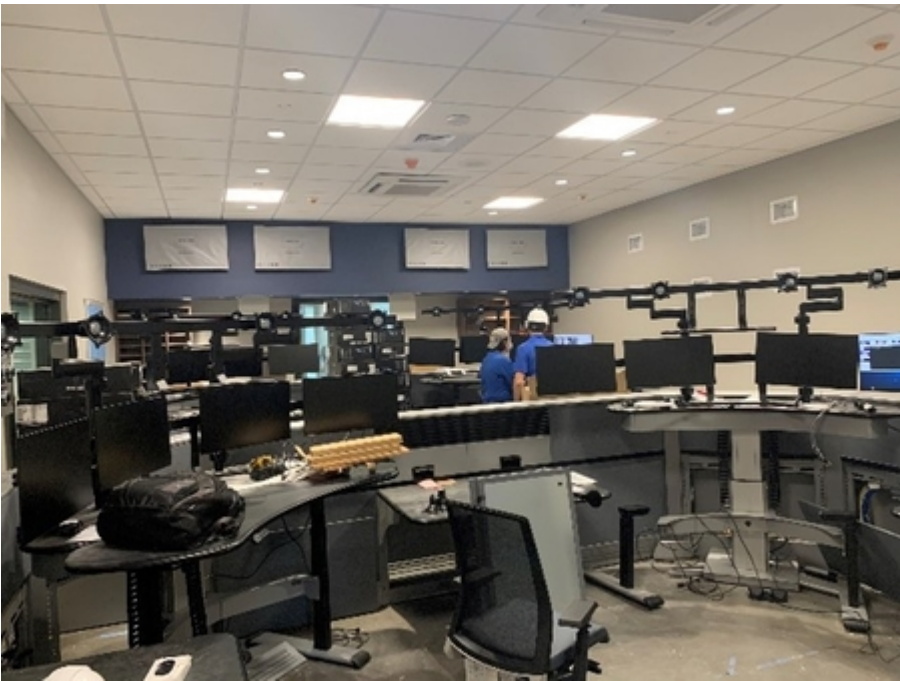
PSC 7/20 Dispatch installation
