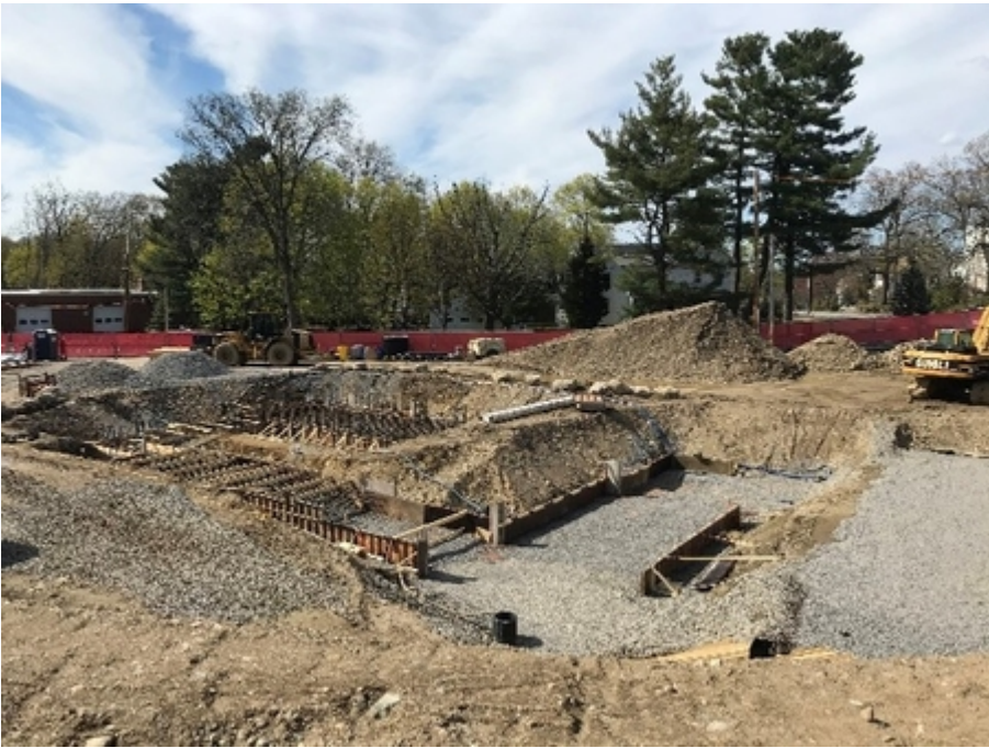
FS#2 4/20 Excavation for FS#2
