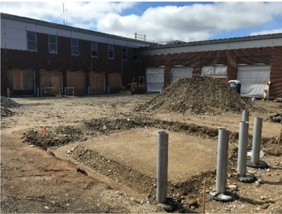
PSC 3/20 View from east ongoing site work
