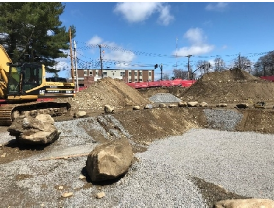
FS#2 3/20 Beginning excavation at FS#2
