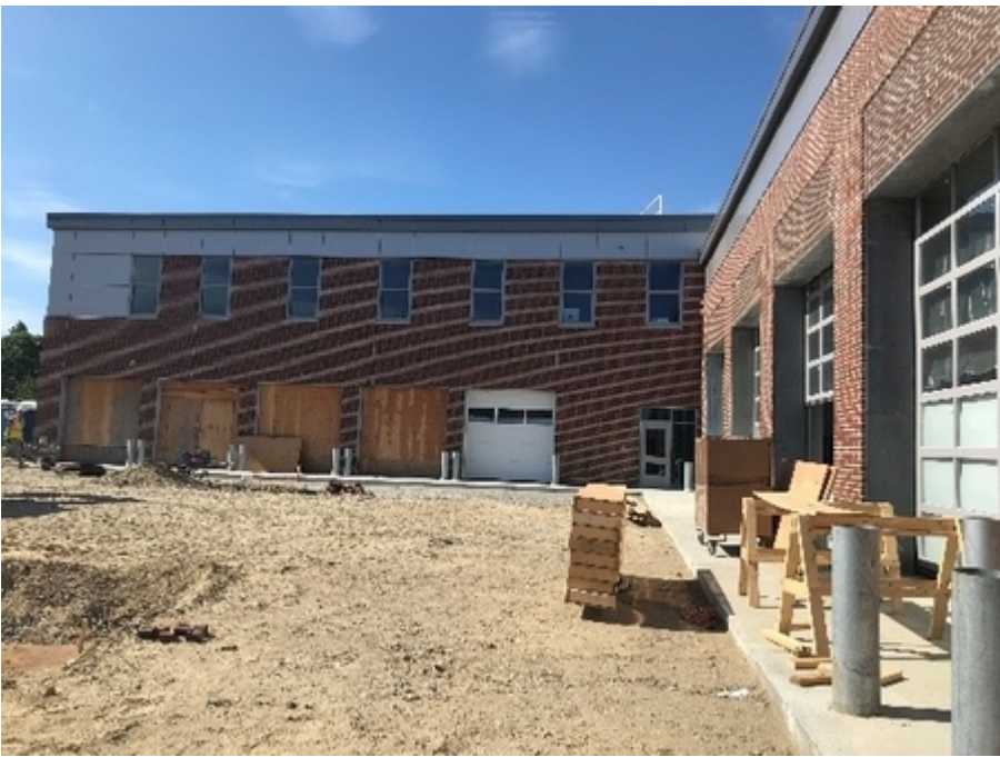
PSC 5/20 Rear garage bays
