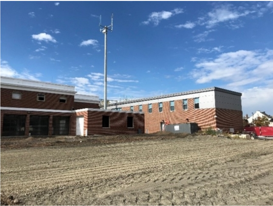
PSC 9/20 Rear elevation with existing old public safety in foreground (on the left)
