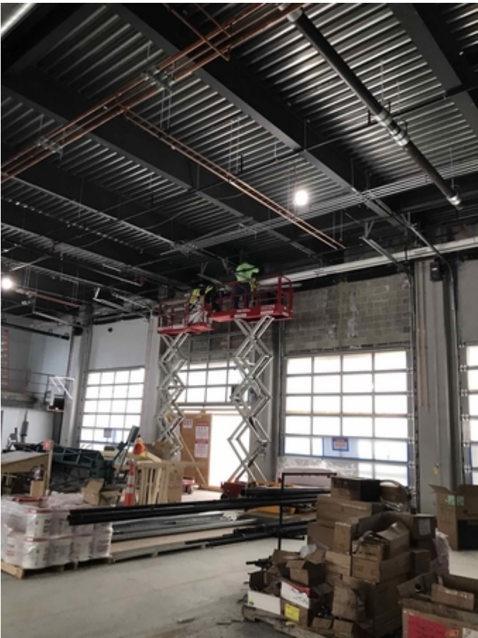
PSC 4/20 Apparatus bay doors installation
