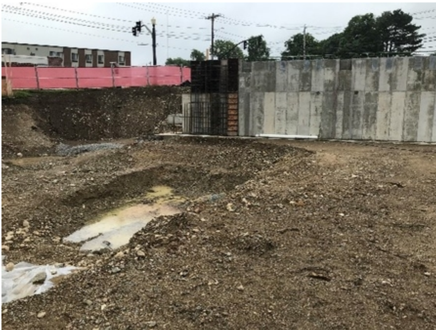
FS#2 6/20 Investigation for contaminated soils
