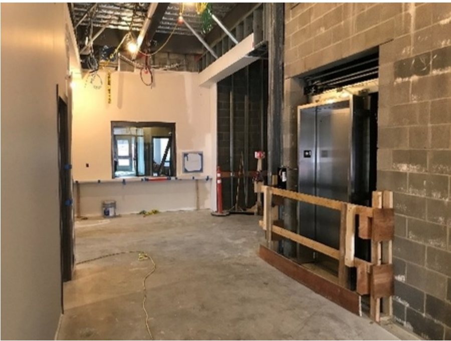
PSC 4/20 Elevator installation
