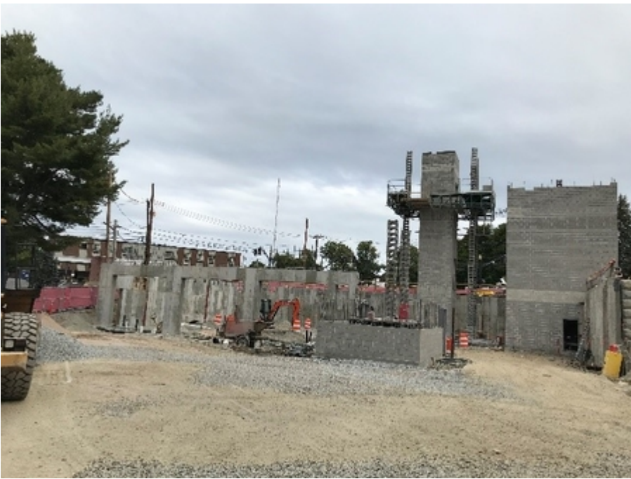
FS#2 9/20 Start of masonry
