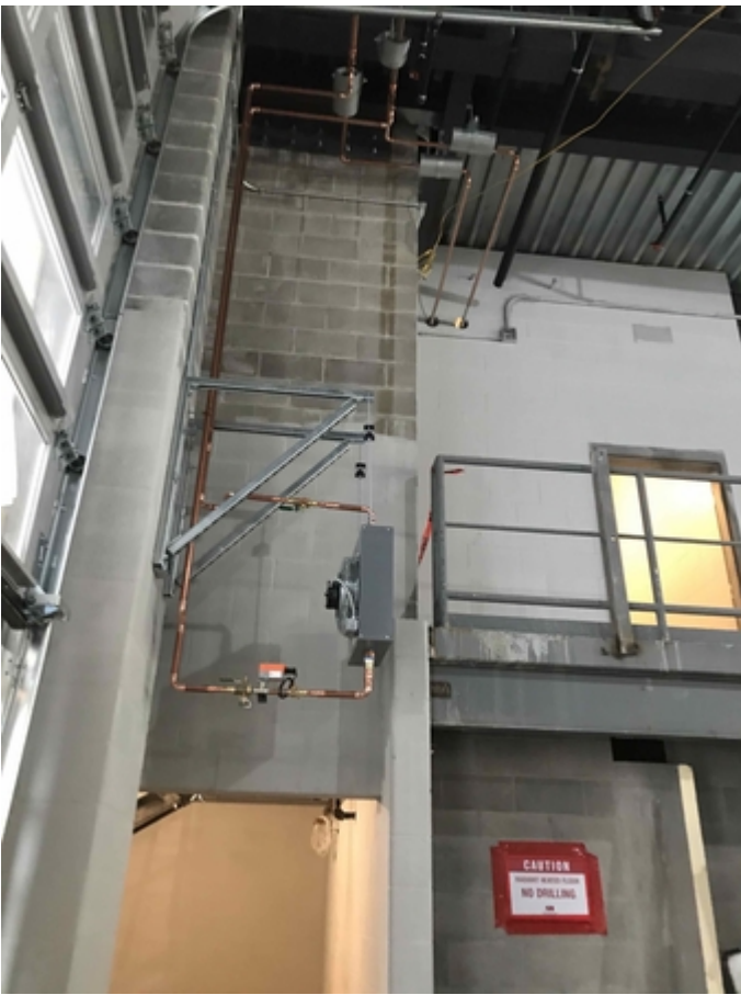
PSC 3/20 Apparatus bay mezzanine area
