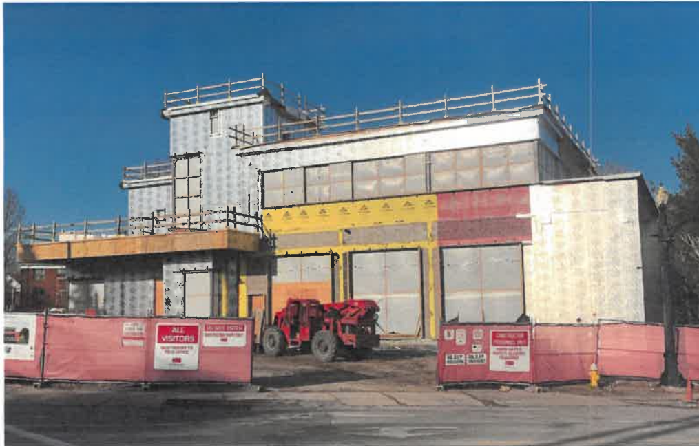
View of front from Webster St
