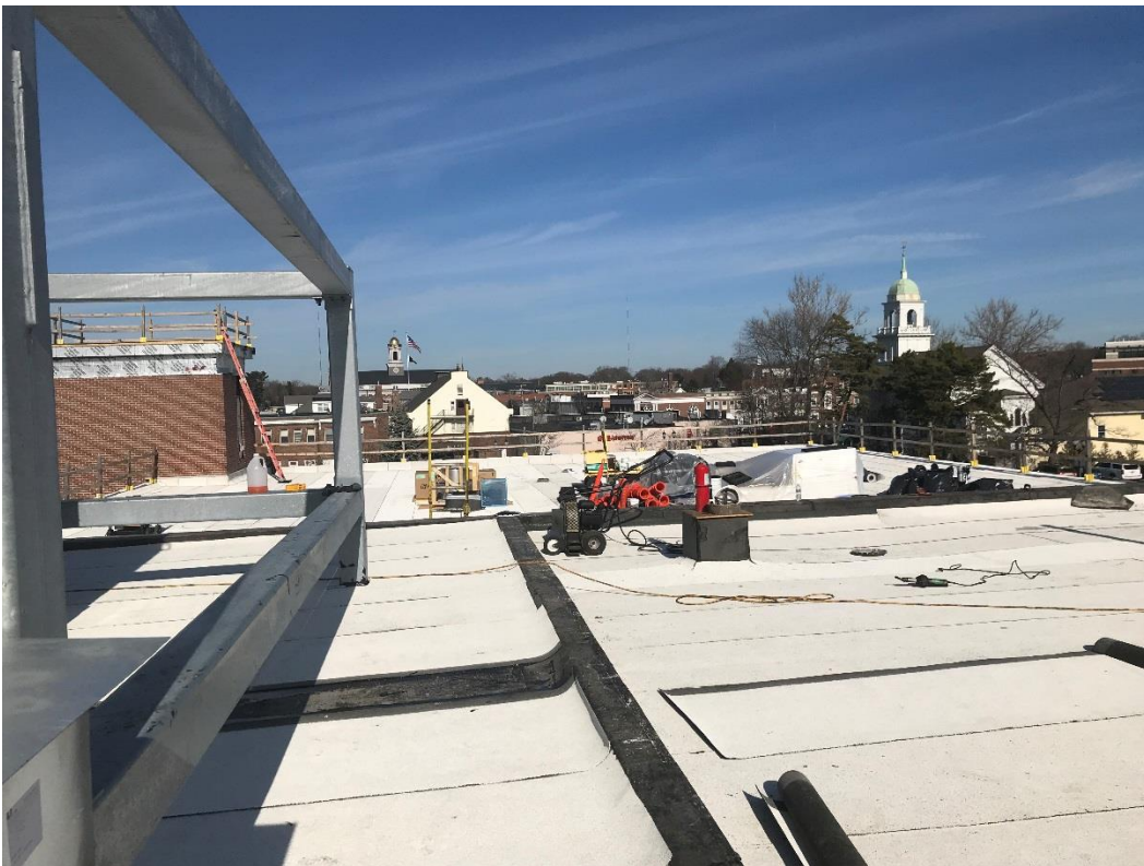
Head Quarters - Fire Station roofing installation
