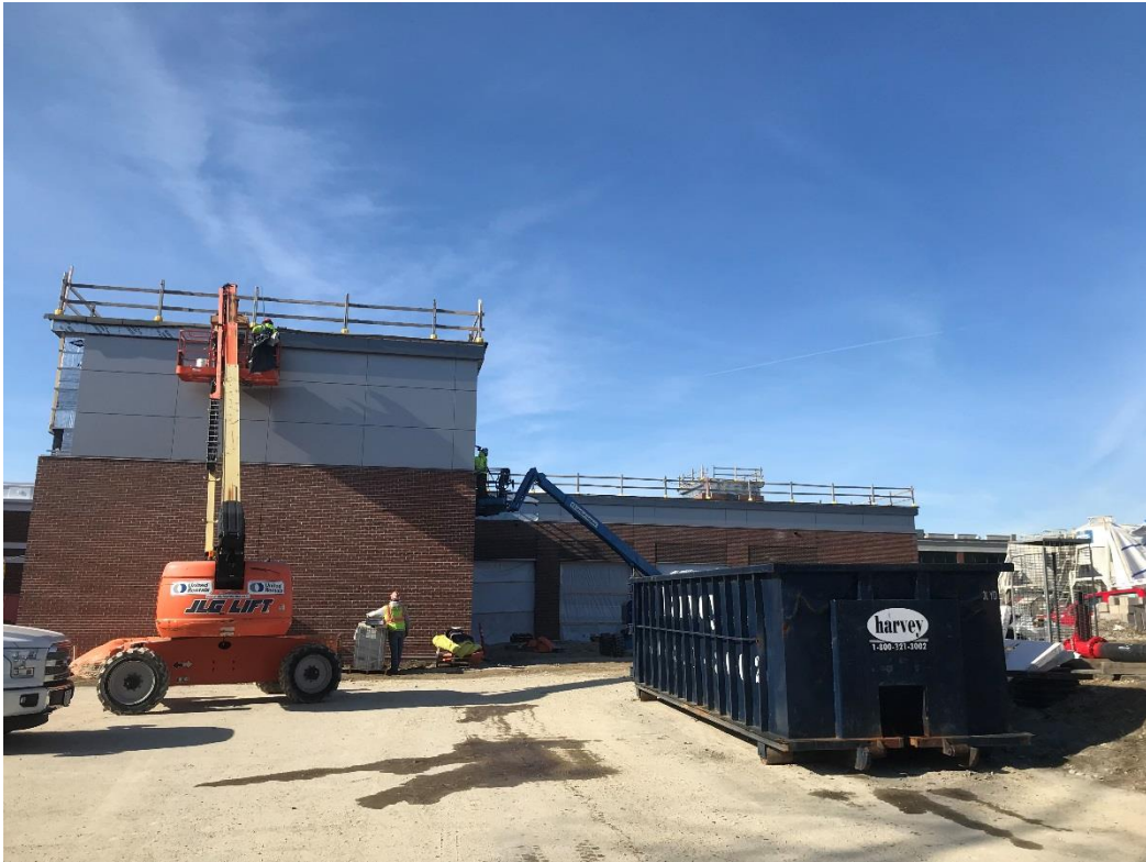
Head Quarters - Fire Station East elevation façade installation
