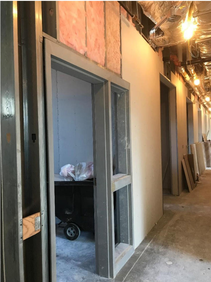
Head Quarters - Fire Station upper level
