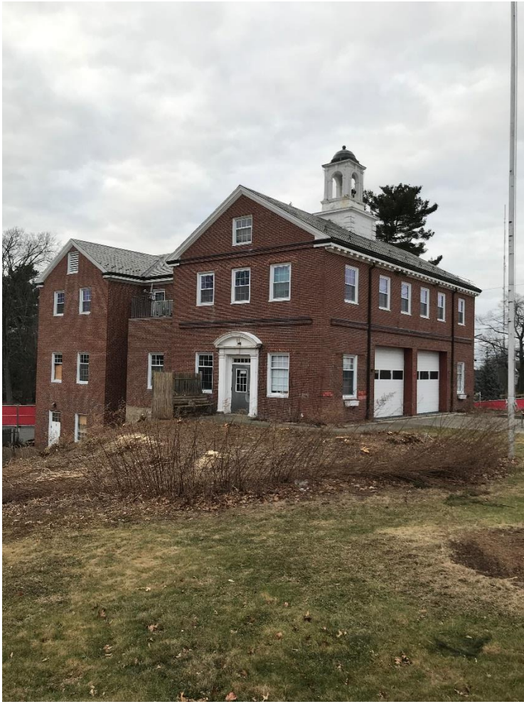
Fire Station #2 Preparing for demolition
