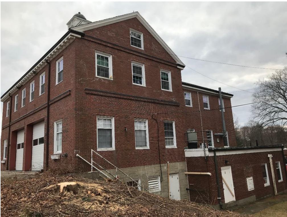
Fire Station #2 Preparing for demolition
