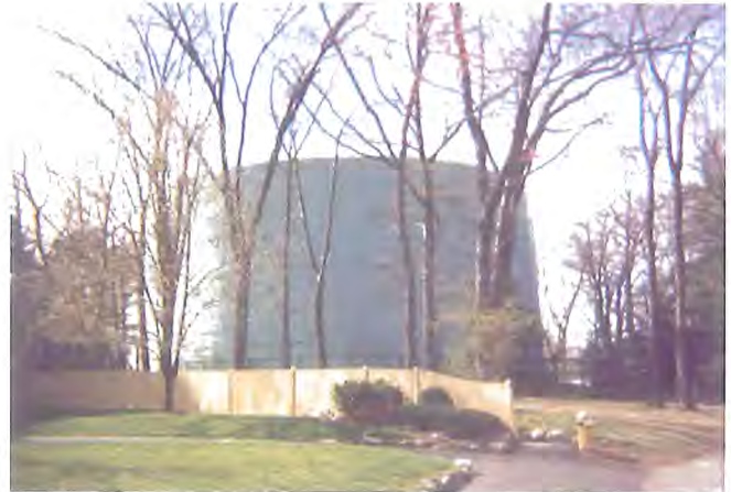
Bird's Hill Storage Tank
