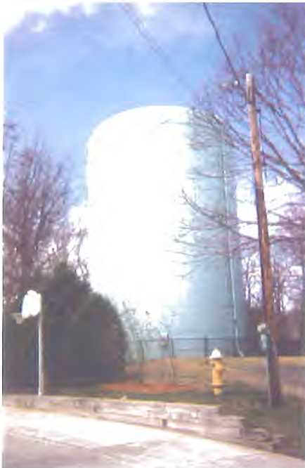
Dunster Road Storage Tank
