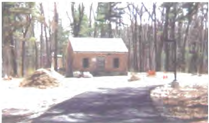
Charles River Wellfield Station No. 3
