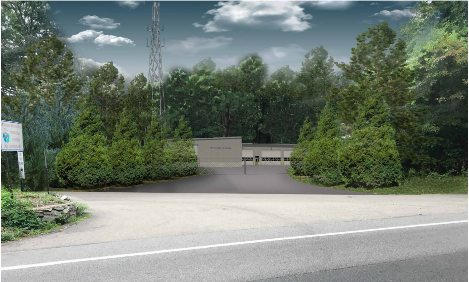
View from RTS driveway
