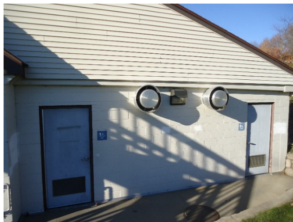
EXISTING EXHAUST FANS SERVING PUBLIC RESTROOMS
