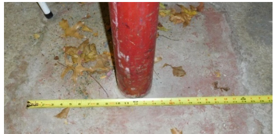
2. Column Foundation and Slab on Grade Patch
