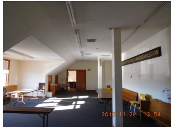
3. SECOND FLOOR COLUMNS SUPPORTING RIDGE
