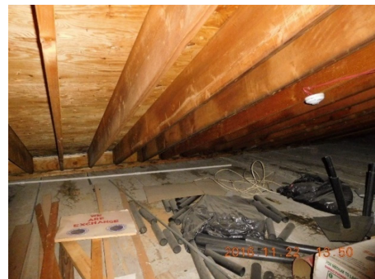
4. ROOF FRAMING AND CONCRETE PLANK ATTIC FLOOR
