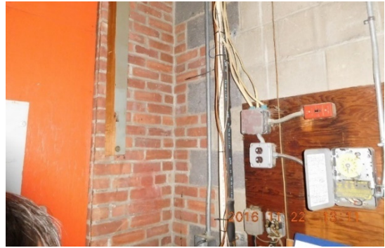
1. Brick and CMU Exterior Walls.
