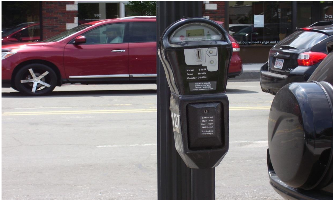
Parking meter and new bracket installed on the new light poles
