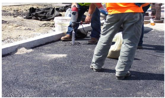
Drilling to construct weep holes in the asphalt base of the brick paver crosswalk
