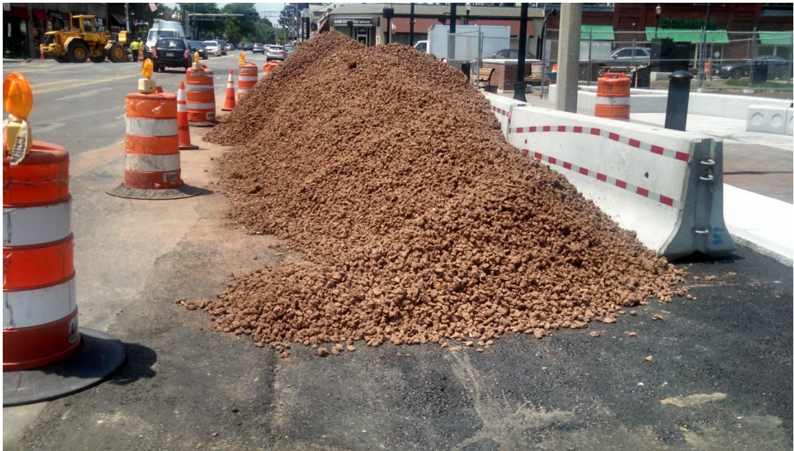
Structural fill for tree planters ready for installation
