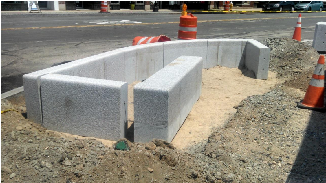
Granite planter with wood seat being installed on the southeast corner of Great Plain Ave. and Dedham Ave.
