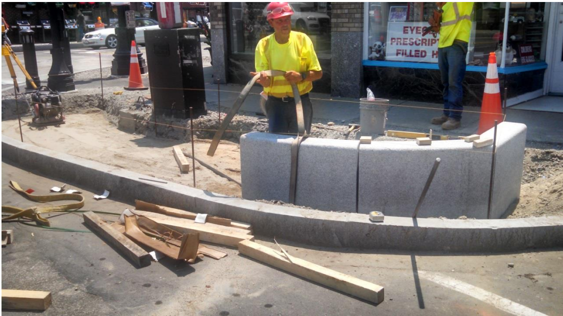
Granite planter with wood seat being installed on the southwest corner of Great Plain Ave. and Chestnut St.
