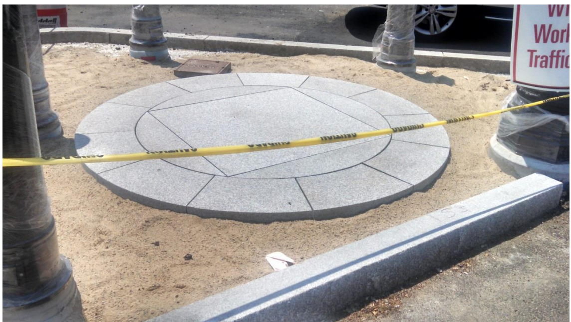
Granite pavers installed for future fountain/sculpture in Dedham Ave. island
