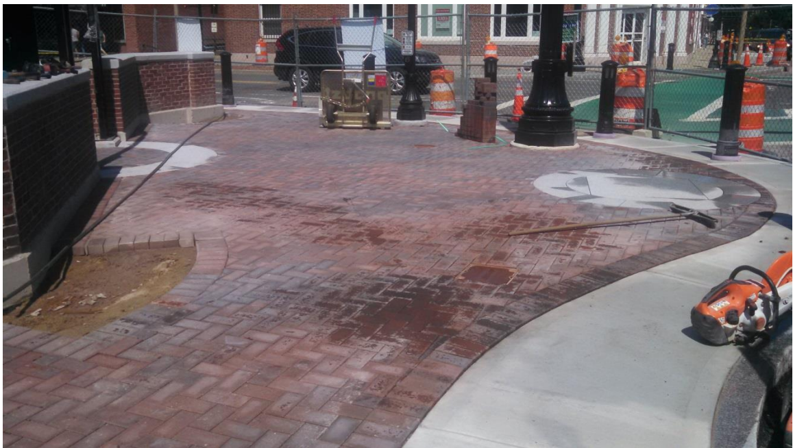
Brick pavers completed at the east end of the Common
