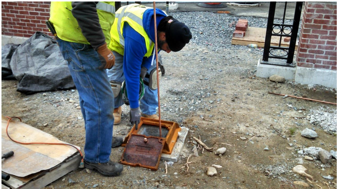
Electricians installing ground rods in hand holes
