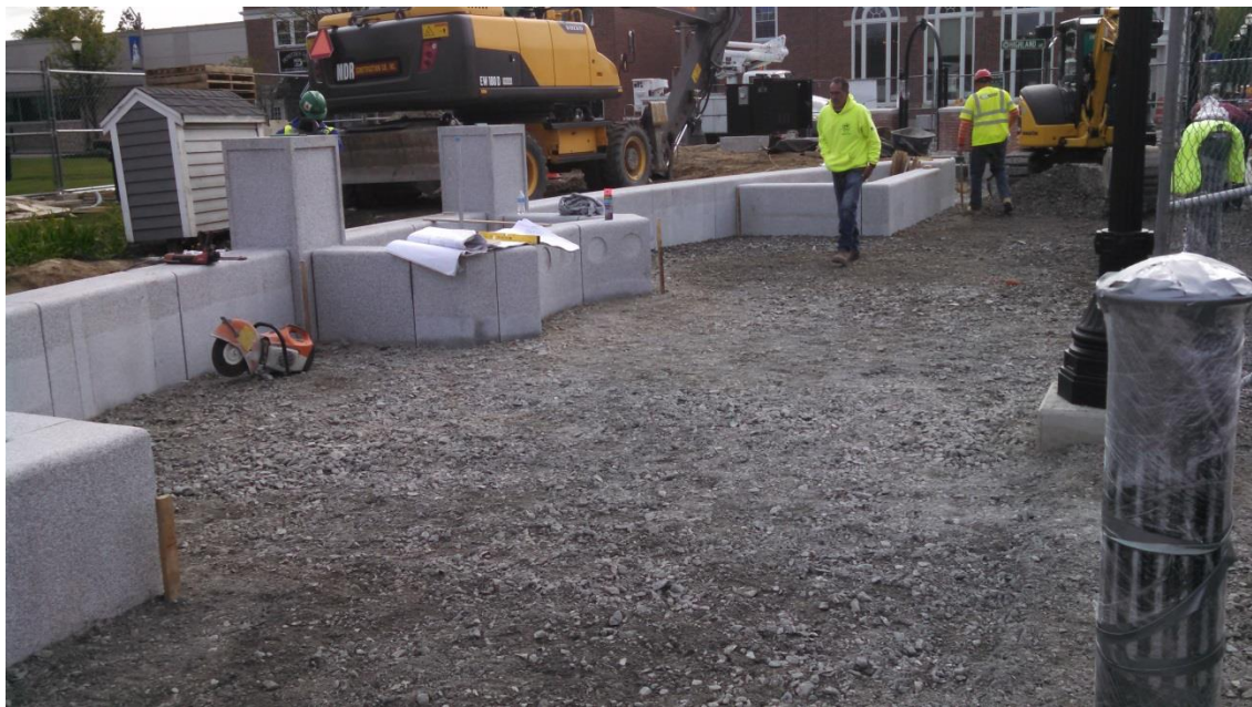
Completed granite seat wall installed in Common
