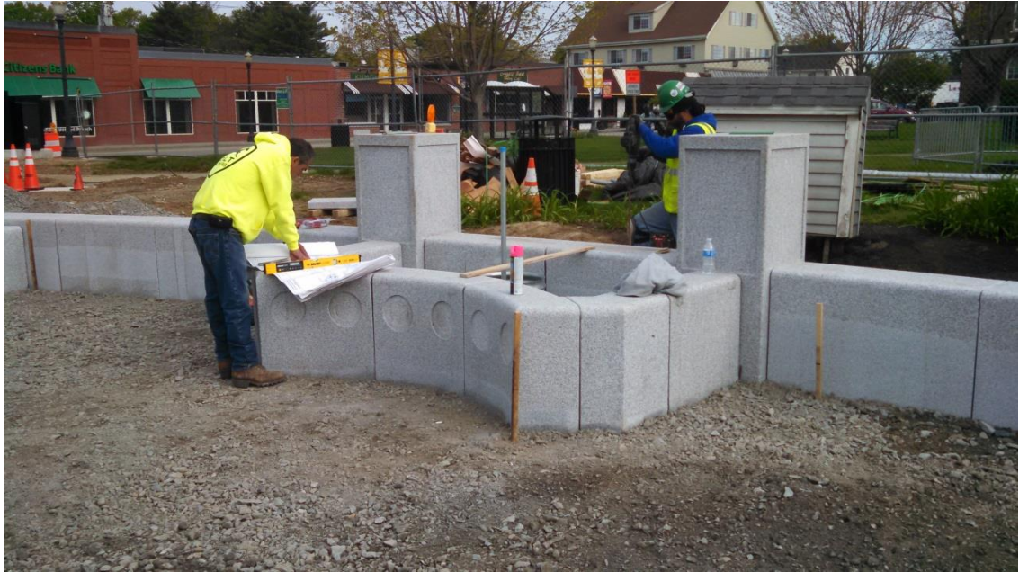
Completed granite seat wall and flagpole planter in Common with electrician installing ground rod in background
