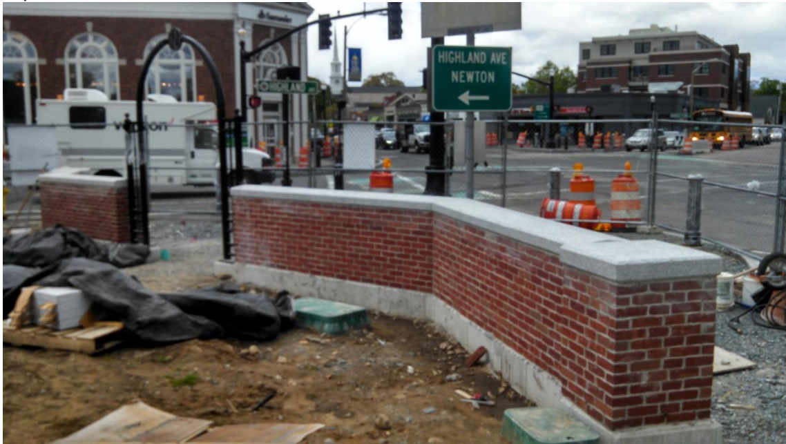
Completed masonry wall with granite capstone at east end of Common
