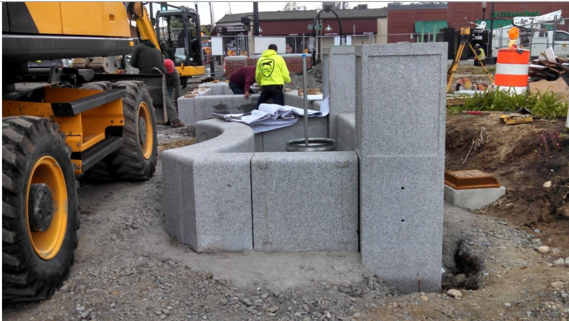
Granite flagpole planter and granite piers with seat wall behind
