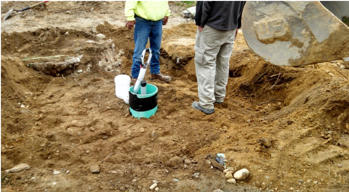
Installation of the base for the new drinking fountain on the west side of the Common
