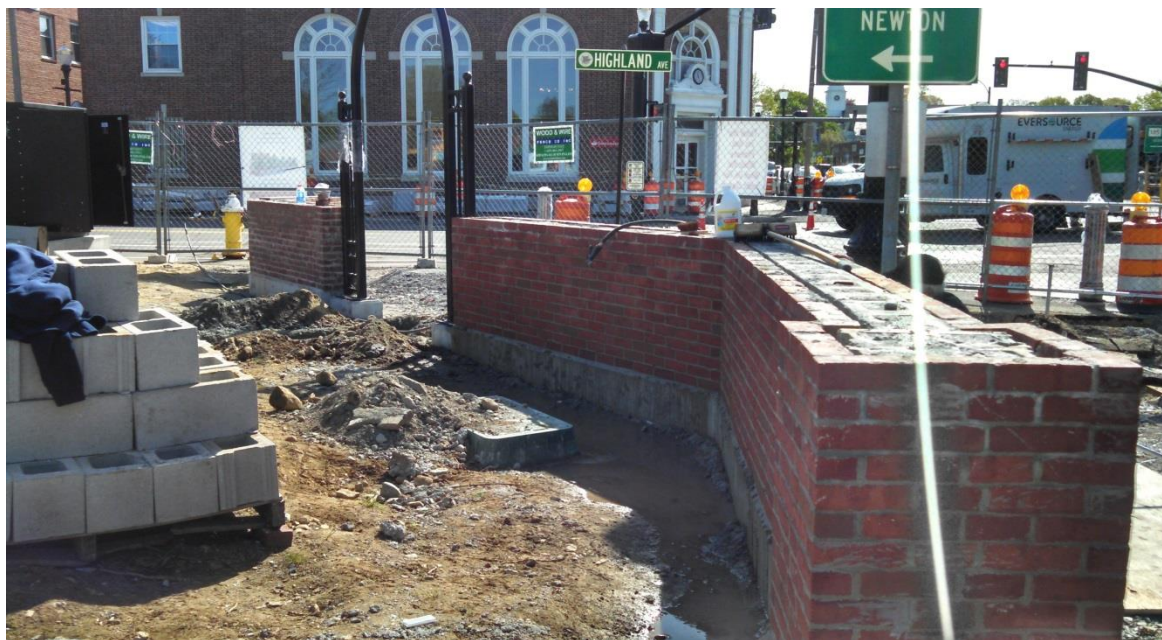
Completed brick masonry wall on the east side of the Common
