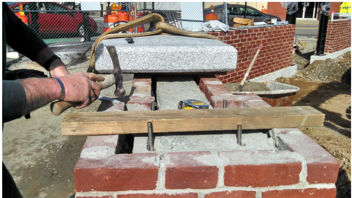
Granite capstone being installed on top of brick masonry wall
