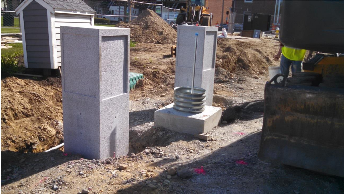
New granite piers adjacent to proposed flagpole foundation
