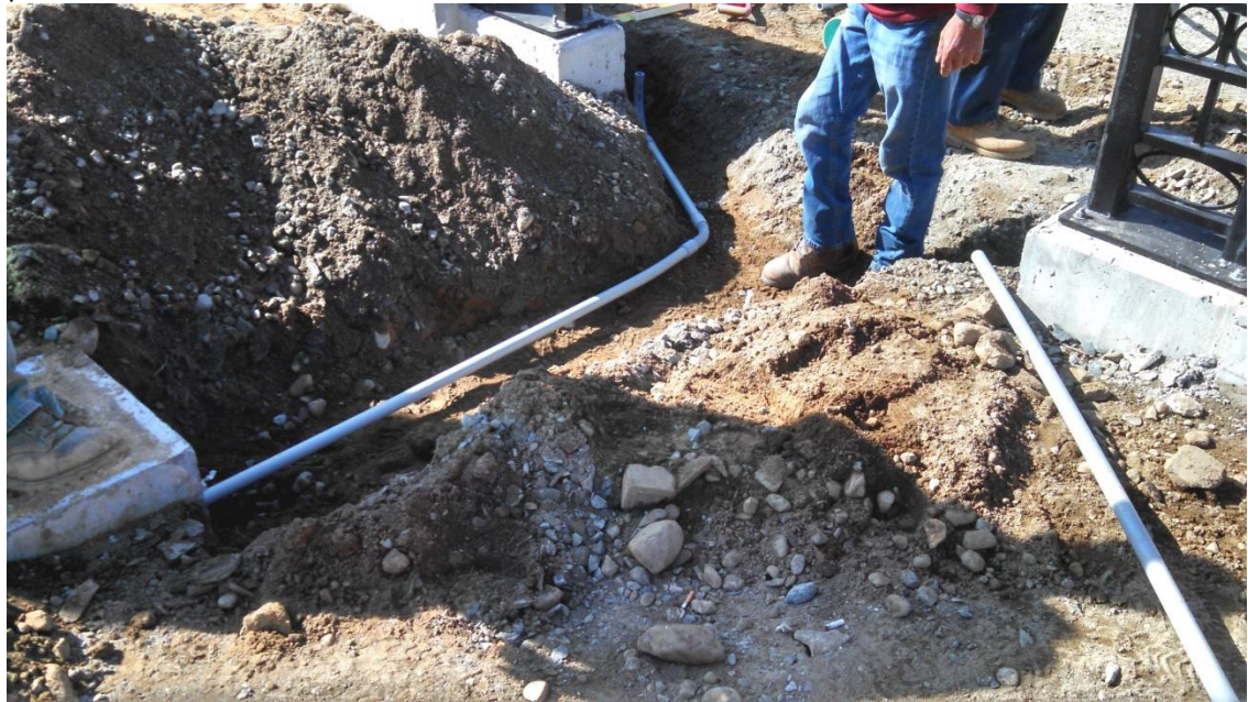
Installing conduit for new up lighting at the ornamental gateway
