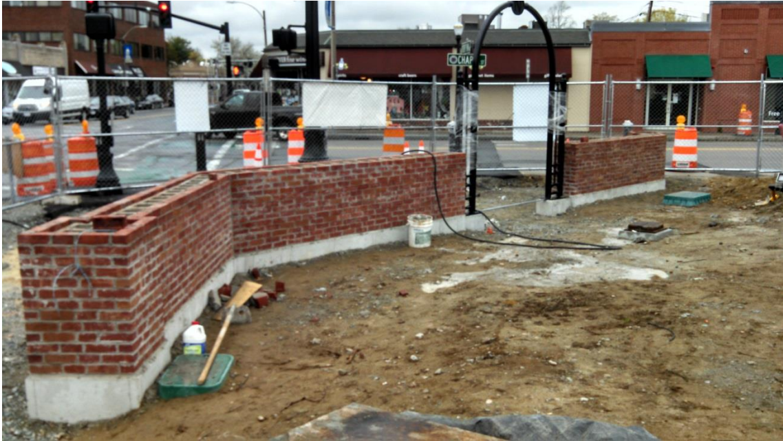
Rear of brick masonry wall completed on the west side Common entrance
