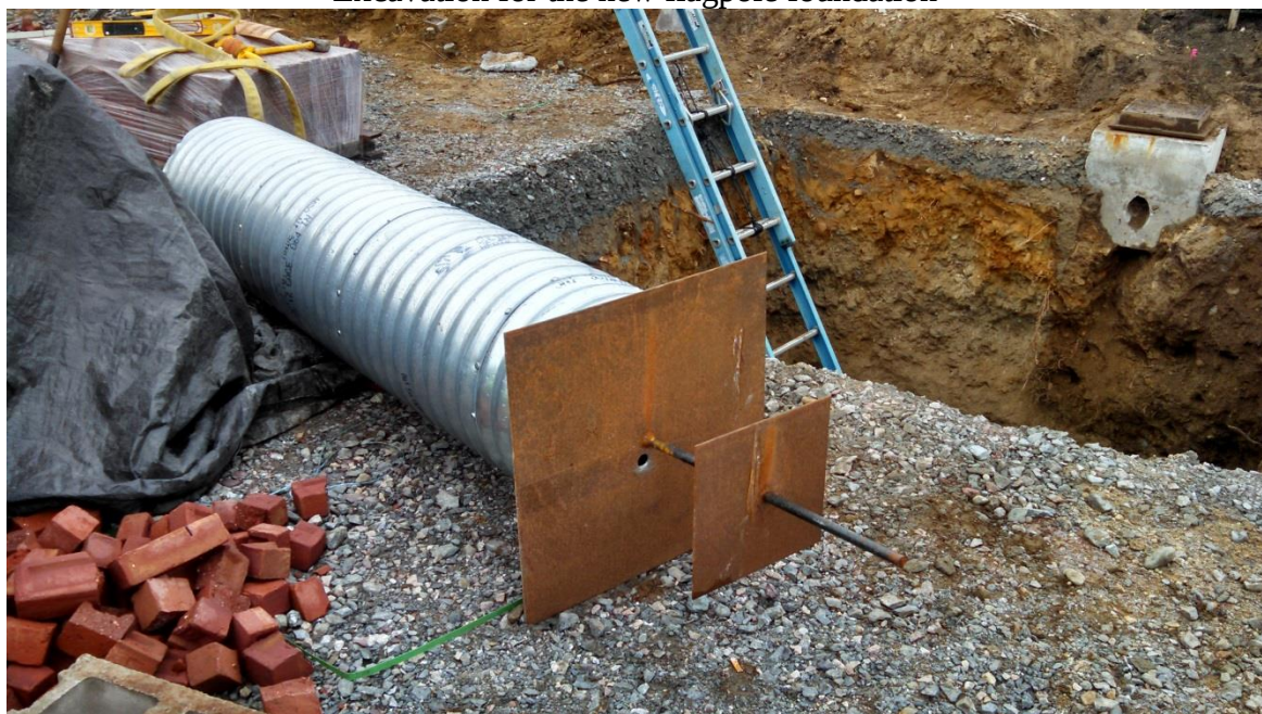
Sleeve and base plate for new flagpole being installed
