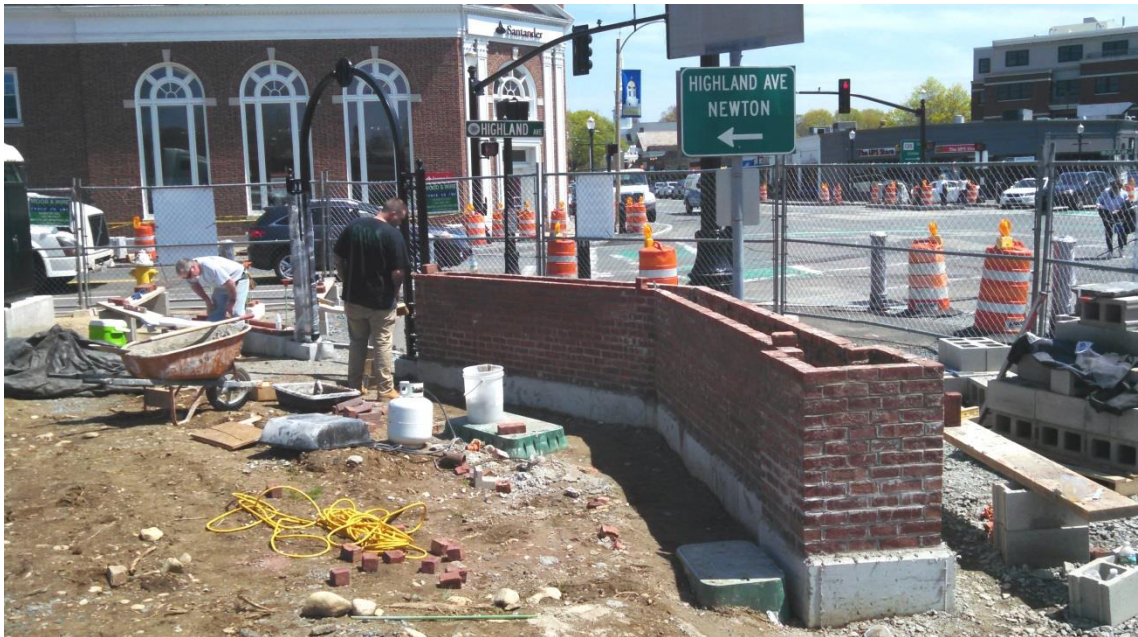
Continued construction of the brick masonry wall on the east side of the Common entrance
