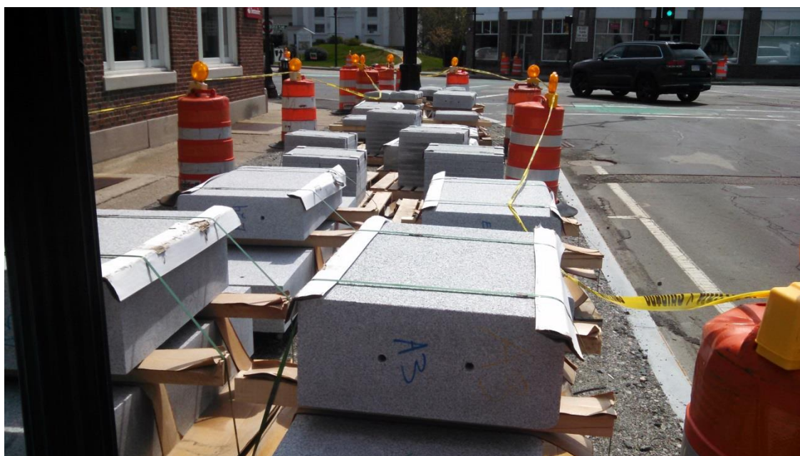
New granite seat wall, pavers and capstones ready for installation
