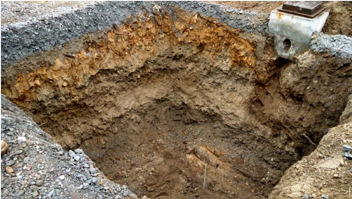
Excavation for the new flagpole foundation
