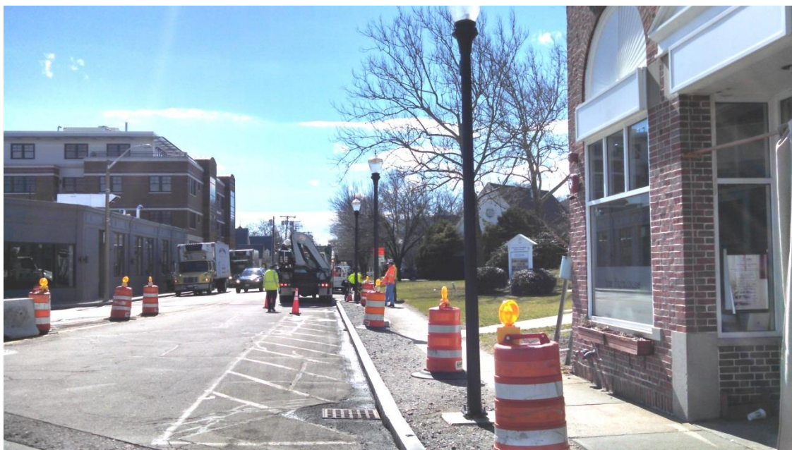
Row of new street lights on the west side of Dedham Ave.
