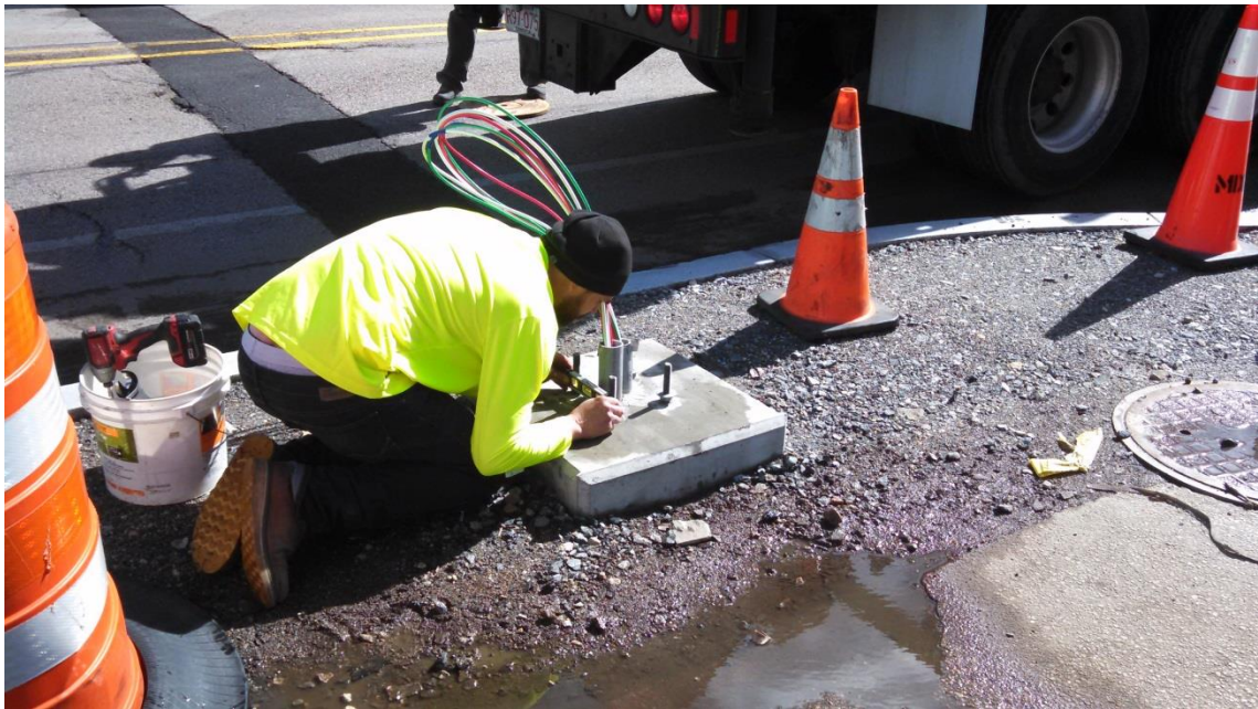
Preparing concrete base for new street light installation on Dedham Ave.
