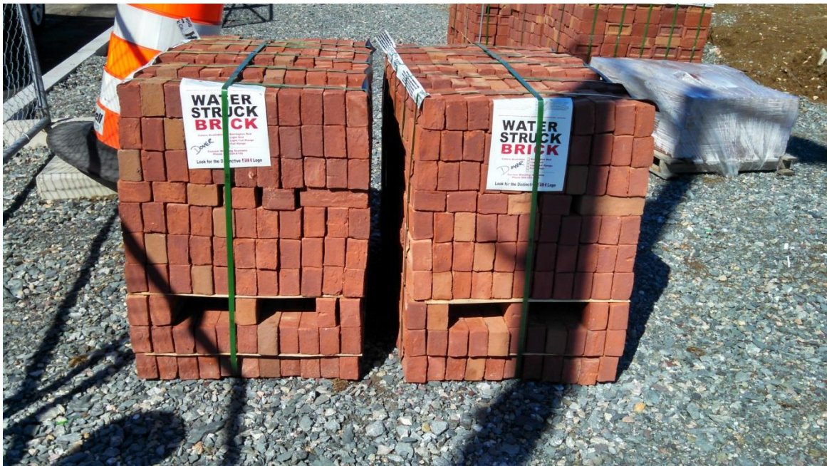
Delivered bricks for construction of the brick masonry wall at the entrance to the Common
