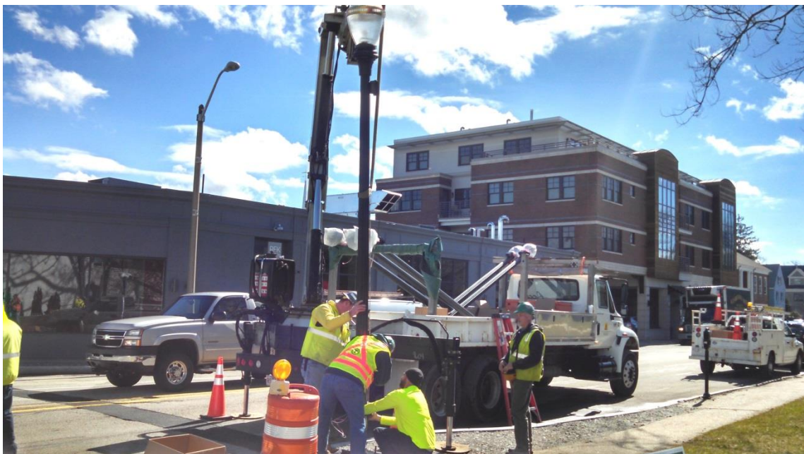
Installing new street light on Dedham Ave
