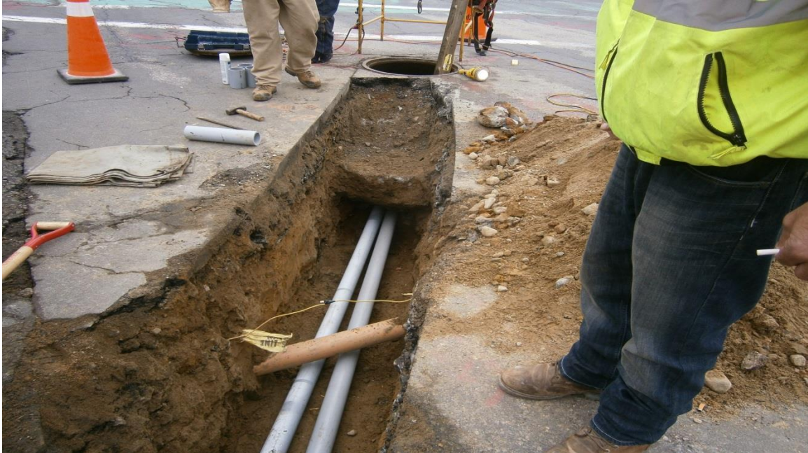
Installing power conduits to the electric vault in Great Plain Ave. at the intersection of Highland Ave.
