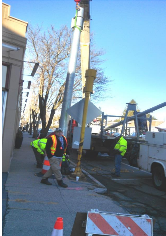
Installing the mast arm pole just west of the train tracks in Great Plain Ave.
