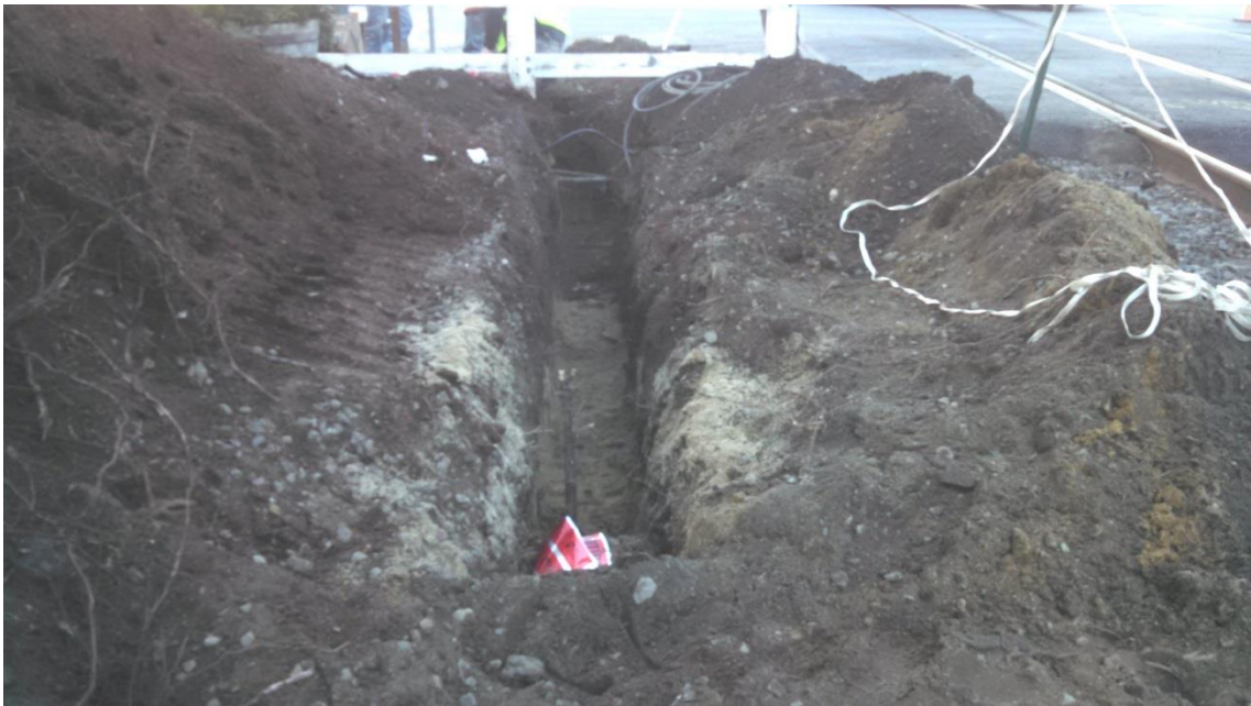
Trench for 3 inch PVC schedule 80 conduit showing sand bedding, warning tape and existing cables near sidewalk
