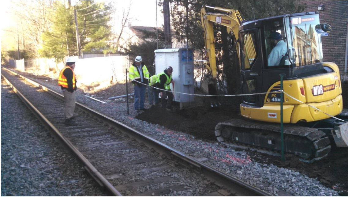
Excavating for installation of 3 inch schedule 80 PVC conduit in MBTA right-of-way with Keolis flagman to the left
