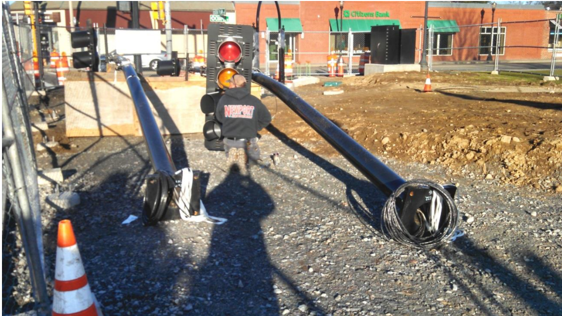
Mast arms being prepped for installation in front of the Common
