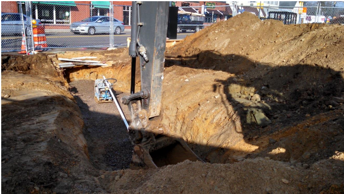
Excavating for the masonry wall foundation footing on the west side of the Common
