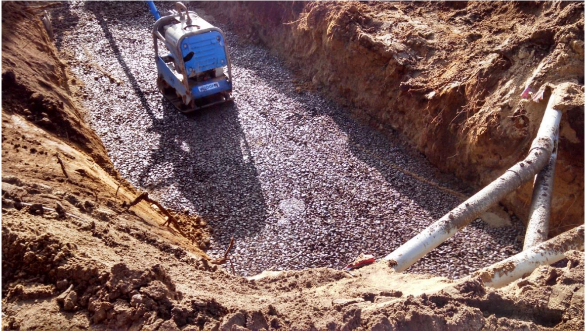
Compacting the sub base for the masonry wall foundation footing on the west side of the Common
