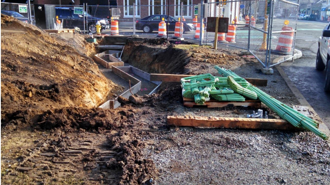
Masonry wall forms for foundation footing on the east side of the Common with reinforcing steel in foreground
