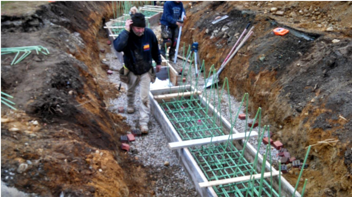
Reinforcing steel installed for the masonry wall foundation footing on the east side of the Common
