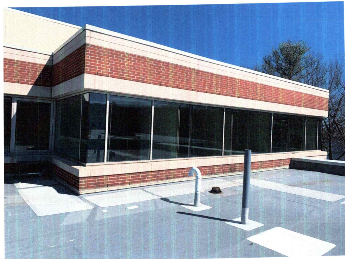
EXISTING VIEW OF ROOF
