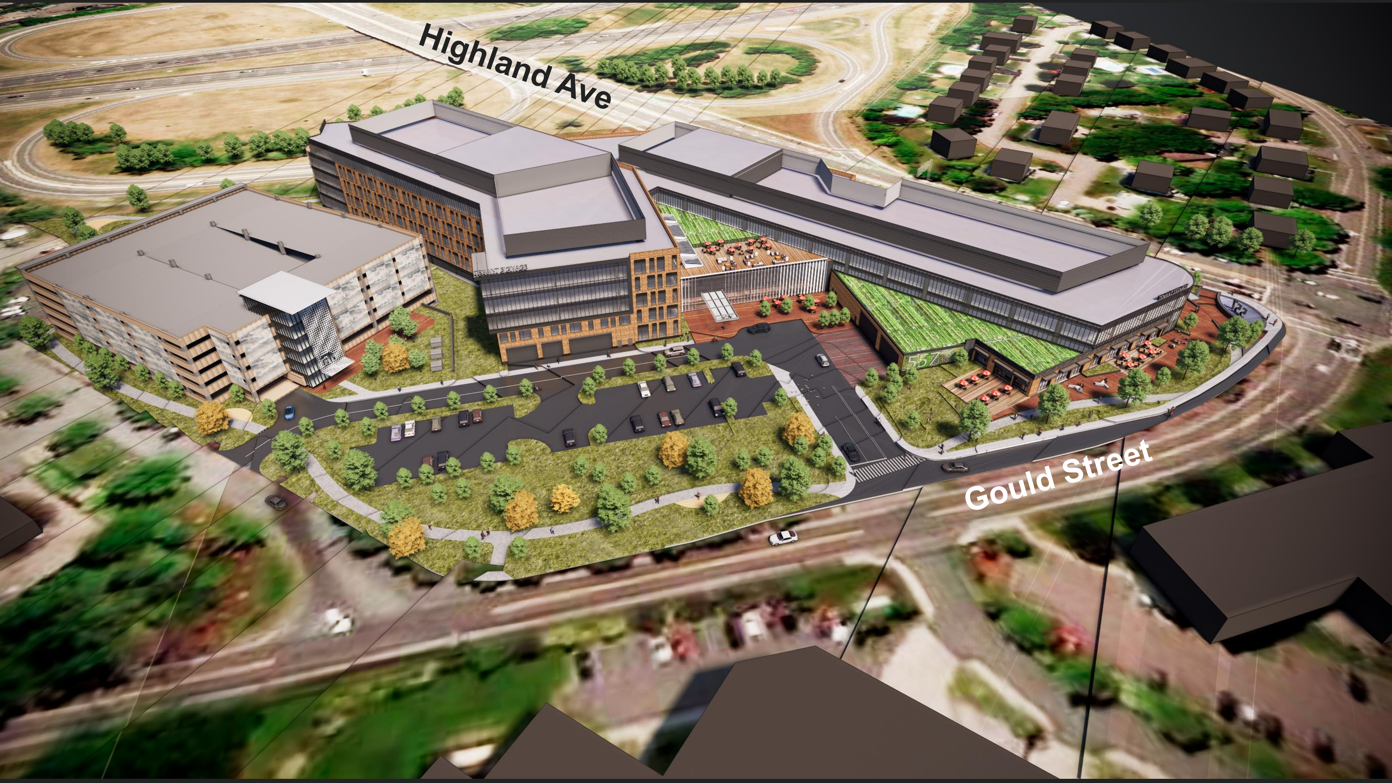
Aerial – Looking North
