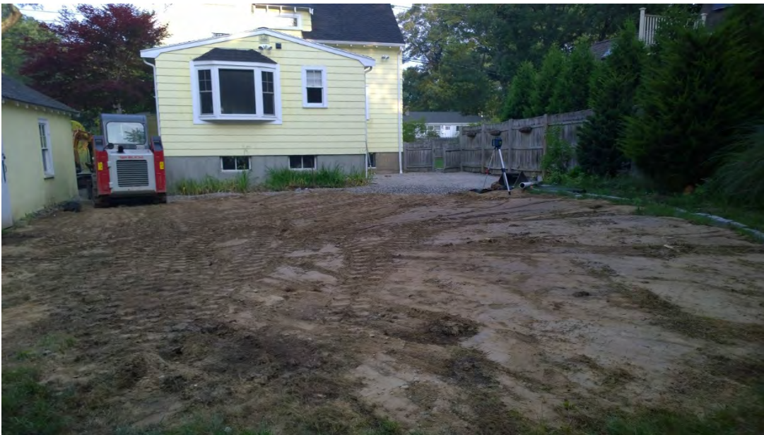
Photo 6: Backyard after subsurface infiltration system installed. Garage on left side of photo. Photo taken July 2015.
