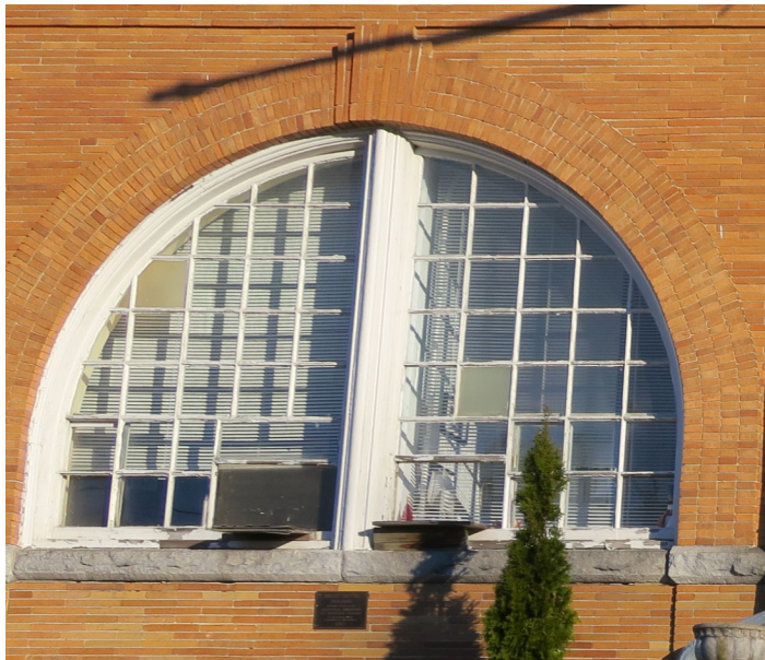
Existing painted wood windows with single glazing
