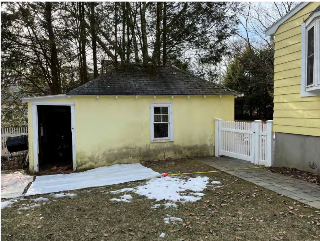
Photo 4: Tarps illustrate location of garage 10 feet behind house. Photo taken on 01/21/22.
