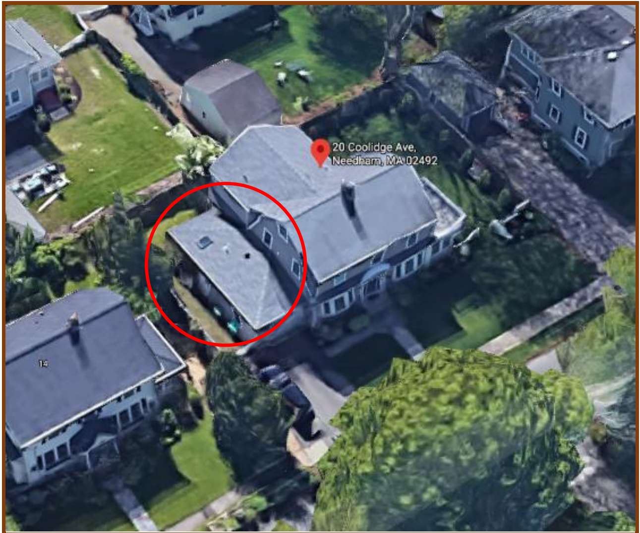
Aerial View – Showing Proposed Location of Work
