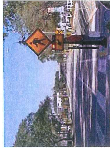
Figure 37: Example Rectangular Rapid Flashing Beacon Installation (FHWA)
