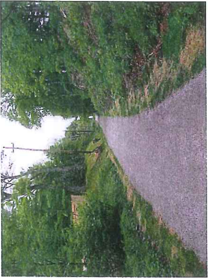
Figure 6: Example Stone Trail Surface Over Dense Graded Crushed Stone Following Construction (Topsfield Linear Common)
