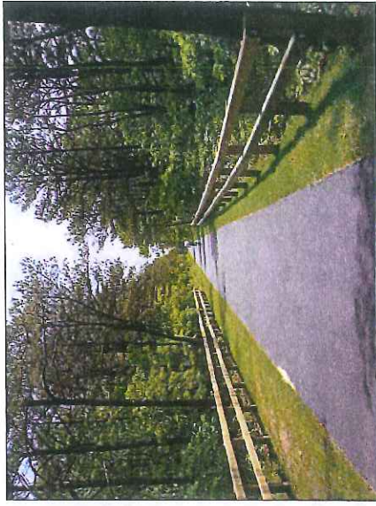
Figure 6: Example Stone Trail Surface Over Dense Graded Crushed Stone Following Construction (Topsfield Linear Common)
