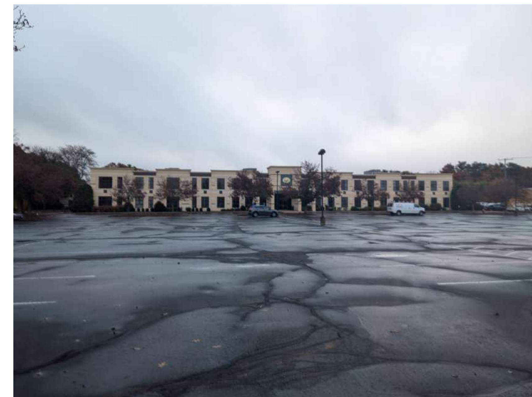
H: NORTH FACE FROM REAR PARKING
