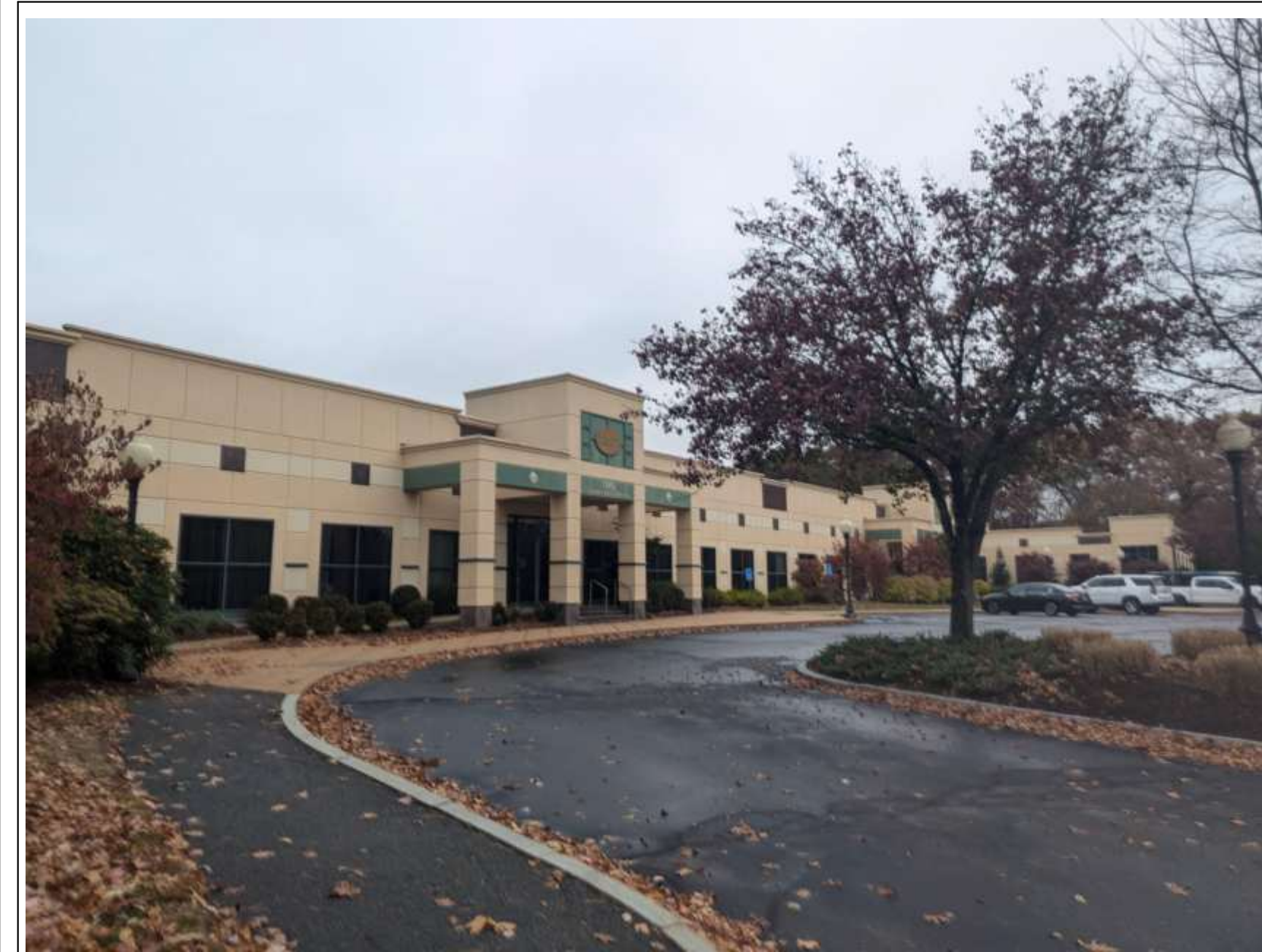
A: SOUTH ENTRY FROM KENDRICK STREET
