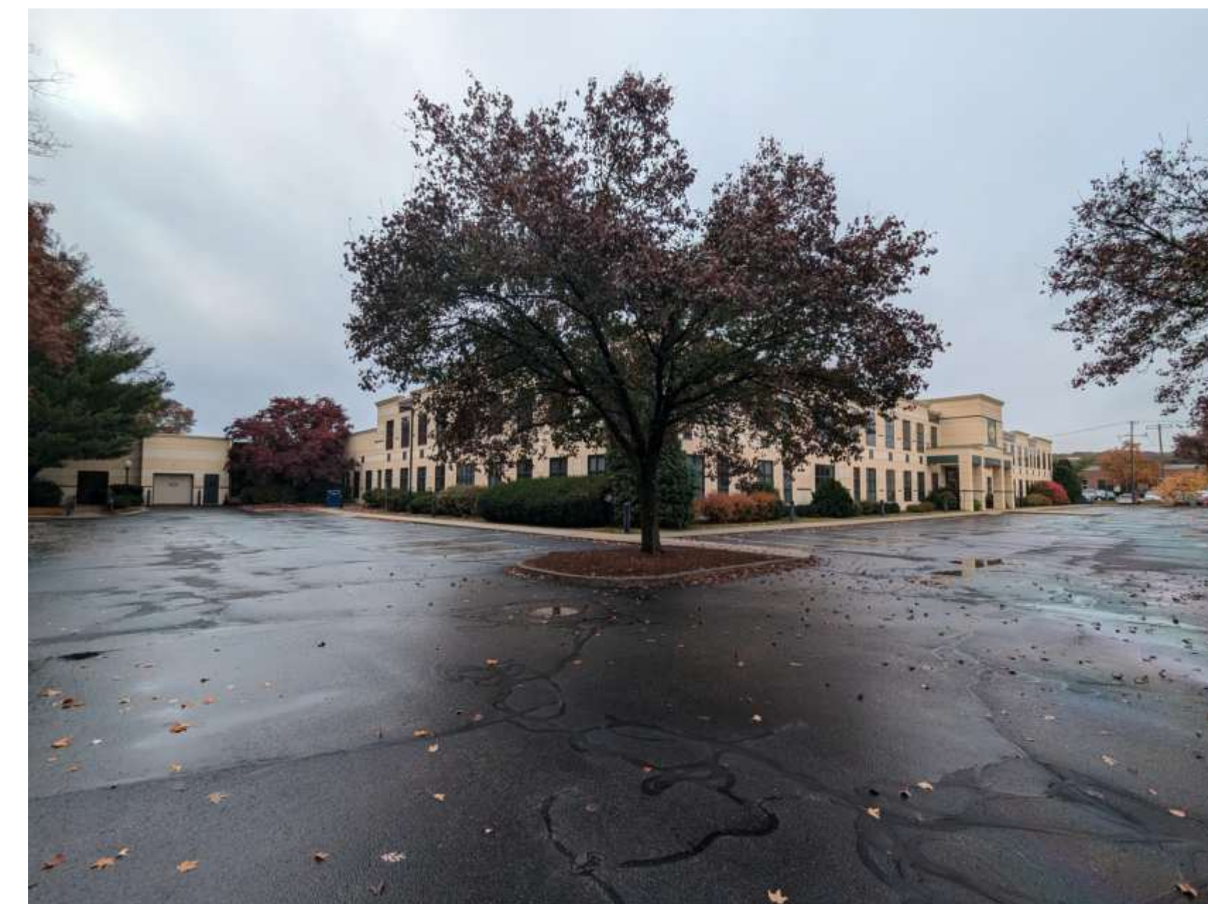
E: NORTH AND EAST FACE FROM REAR PARKING
