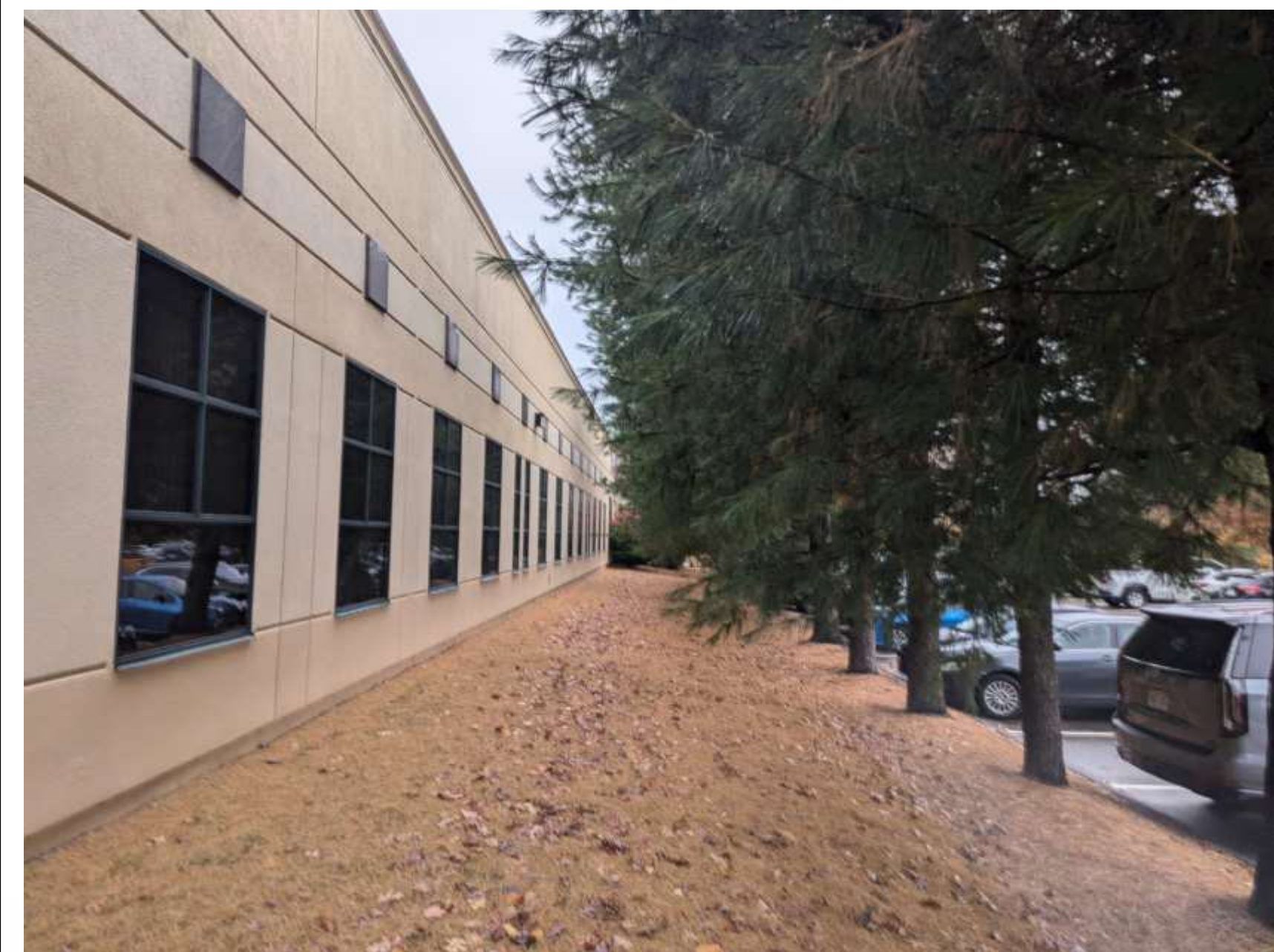
F: WEST FACE OF THE BUILDING
