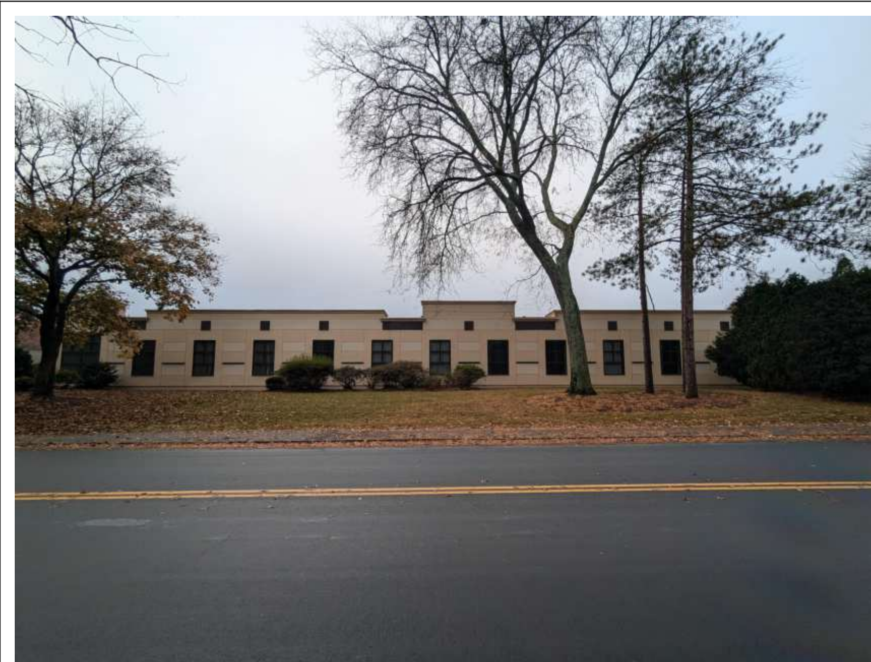
C: EAST FACE OF THE BUILDING FROM 4TH AVENUE
