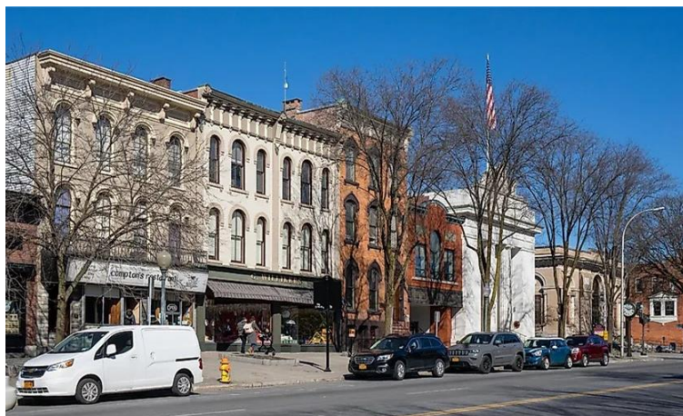
2-3 story MXU multifamily
