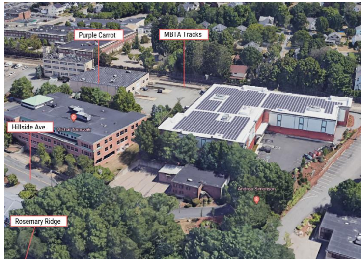
Figure 21: Hillside Industrial District – Base Compliance
