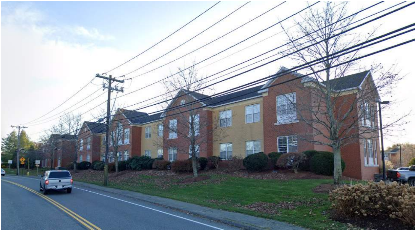
Gould Street Looking South
