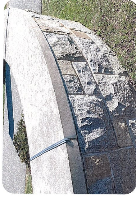
STONE VENEER WITH PRECAST CAP
